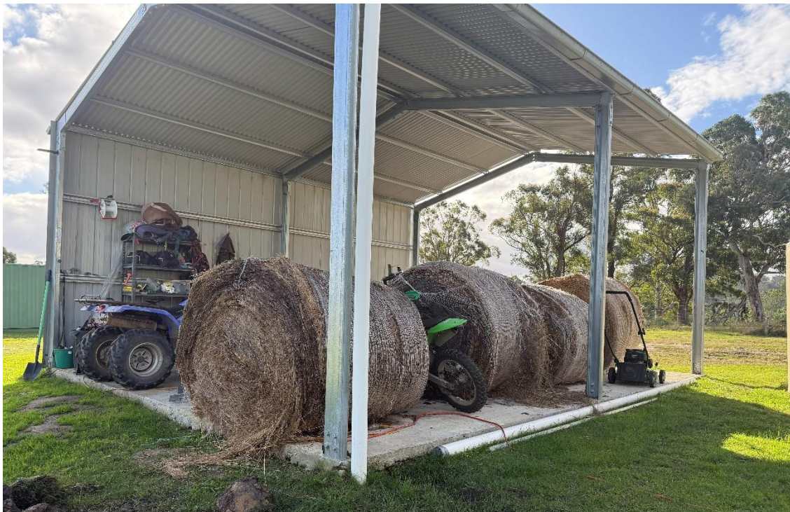
Existing Hay Shed
