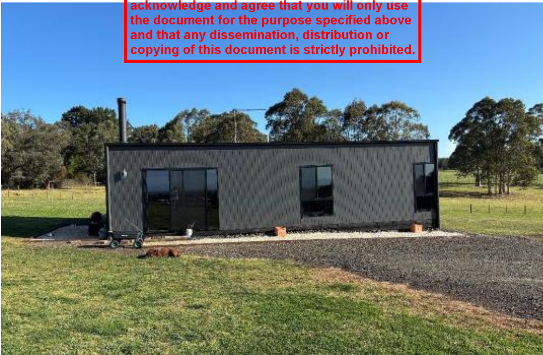
Photograph 3: Existing second dwelling
