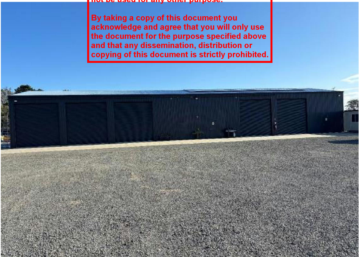
Photograph 1: Existing machinery shed and hardstand
