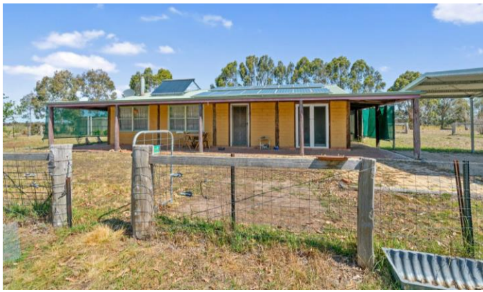
VIEW OF THE CROSSOVER FROM BRADLEYS ROAD TO THE DWELLING ON THE SUBJECT SITE
