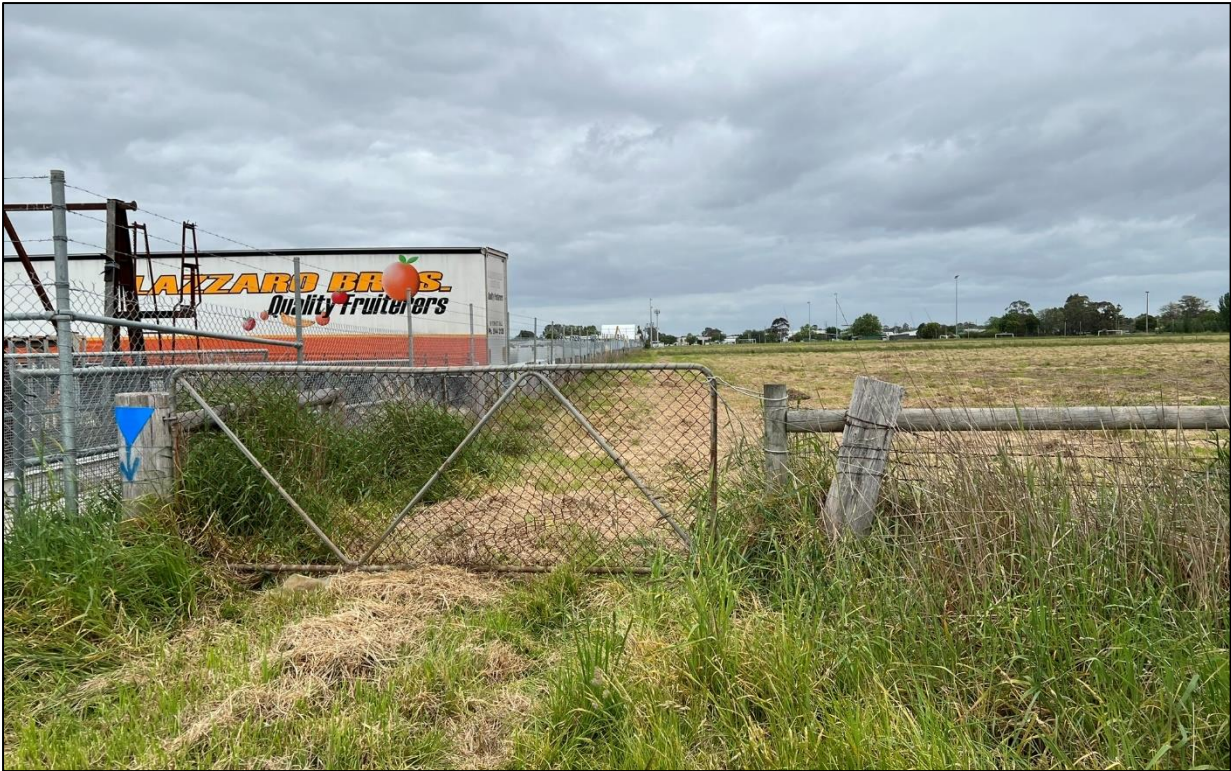
Figure 4: View of the existing site access from Dawson Street looking south
