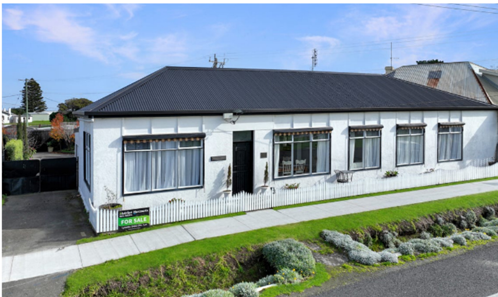
Figure 8: Neighbouring residential building to the east (3 Wharf St)
