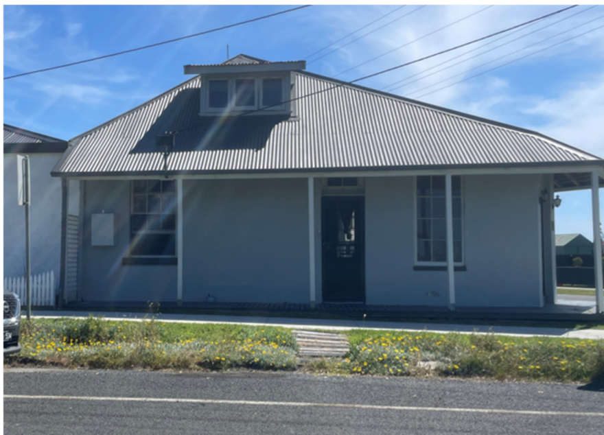
Figure 6: Wharf Street facade
