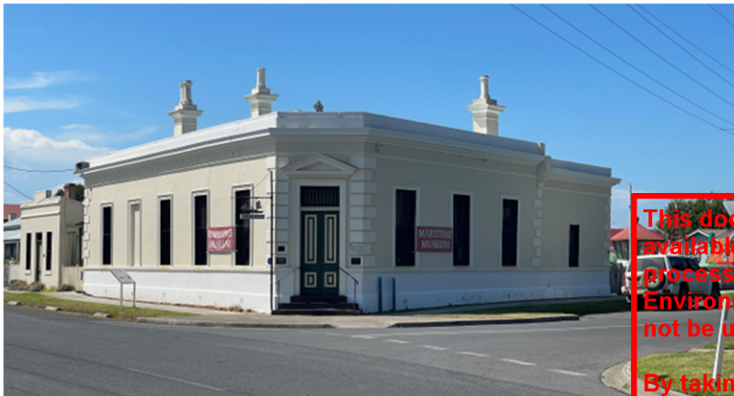
Figure 15: Maritime Museum diagonally opposite the intersection
