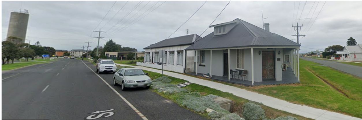
Figure 13: View along Wharf St Map showing Port Albert Heritage Precinct shaded in purple
