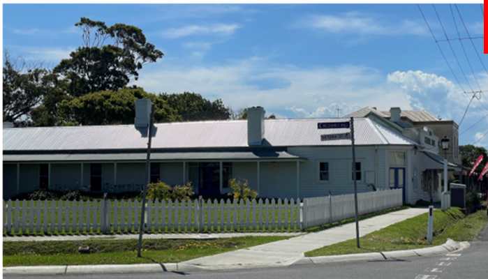
Figure 16: Building across Victoria Street (73 Tarraville Road)
