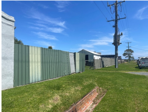
Figure 10: Existing fence on Victoria Street
