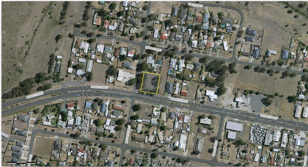
Figure 2: Far aerial showing the site and surrounds.
