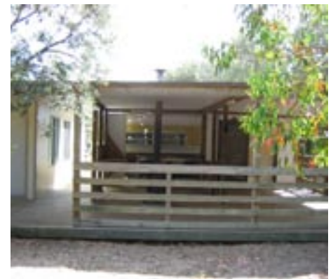
Permanent structure in the camping area
