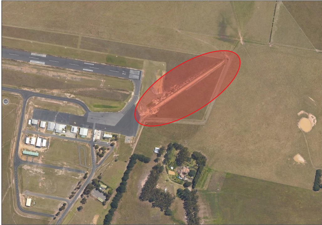
Figure 23: Open stormwater drain
