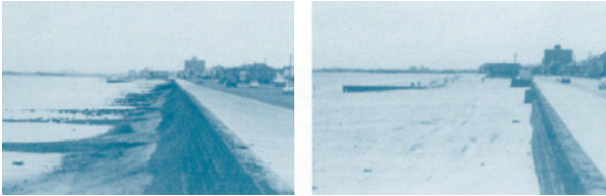
Urban development which has required protective walling and later beach restoration
