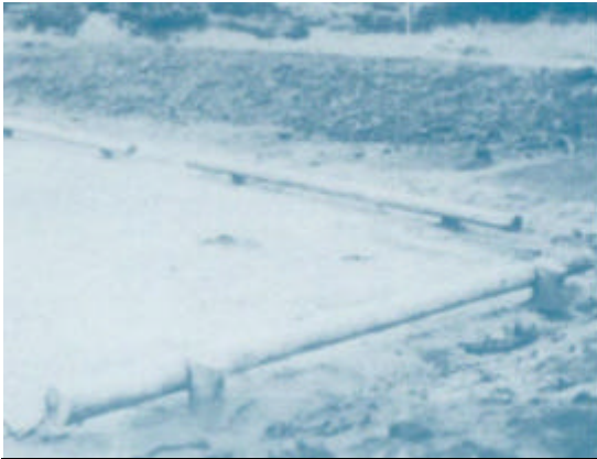
Unobtrusive, low, well constructed pine log vehicle barrier.
