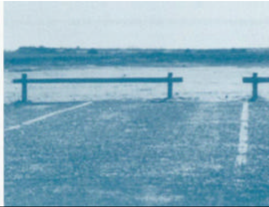
Visually obtrusive pine log vehicle barrier installed too high and with rough detailing
