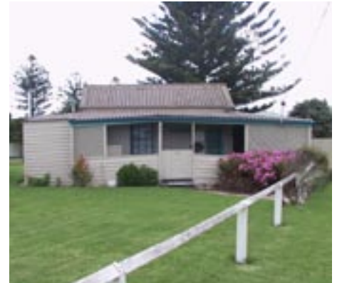
Seaspray cottage near foreshore
