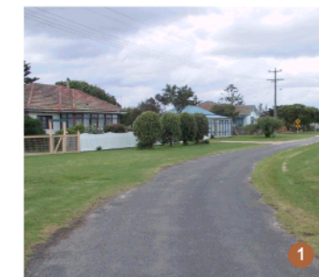
Typical house & road
