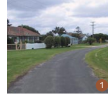
Typical house & road
