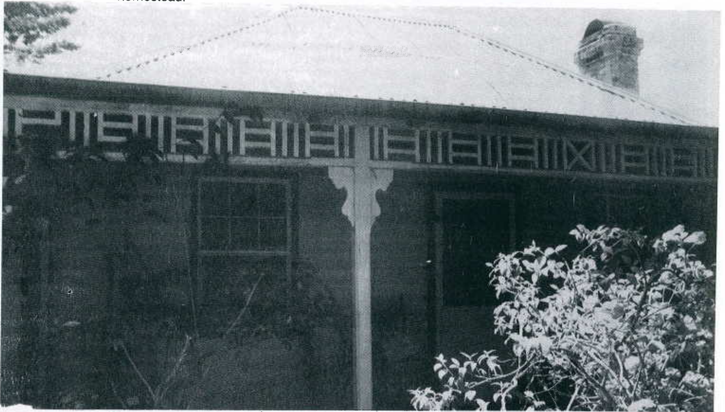
■ 58: Green Hills. West Wing: east elevation, verandah added c1920
