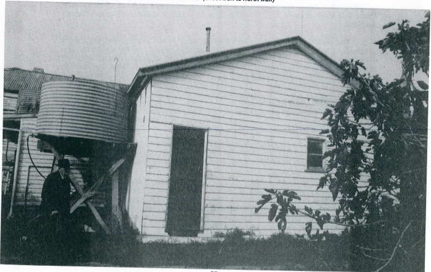
■ West elevation, iron framehouse (sheet iron to north wall)
