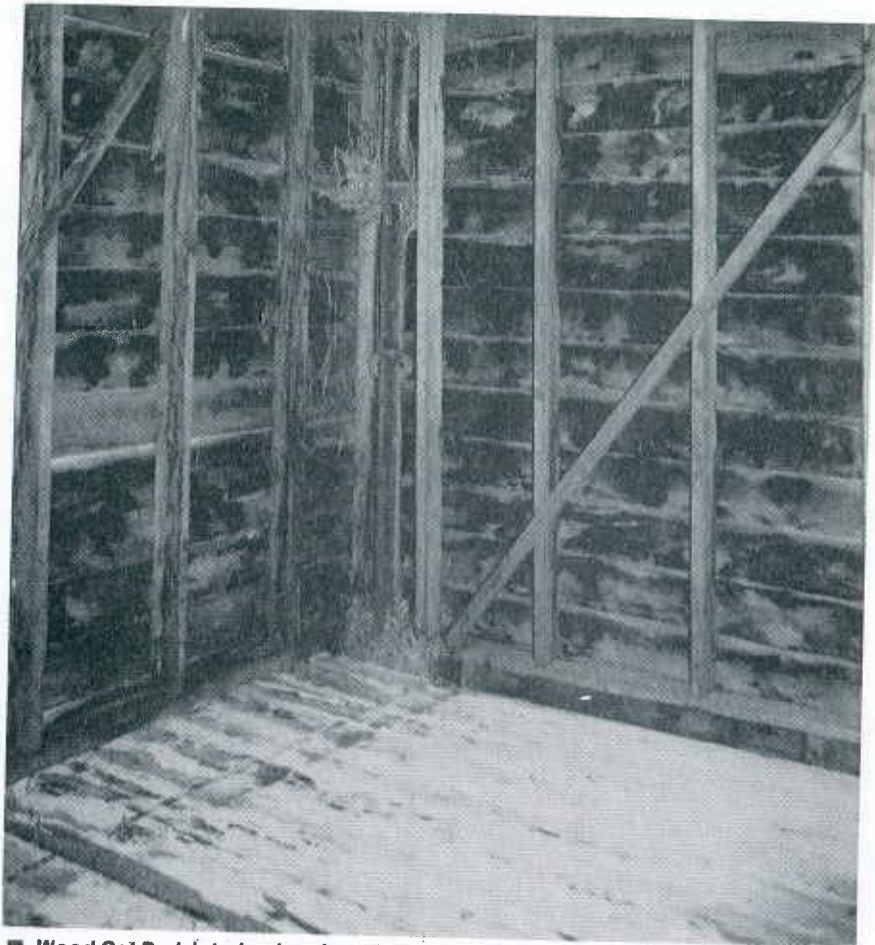
■ Wood Cot Park interior, iron framehouse
