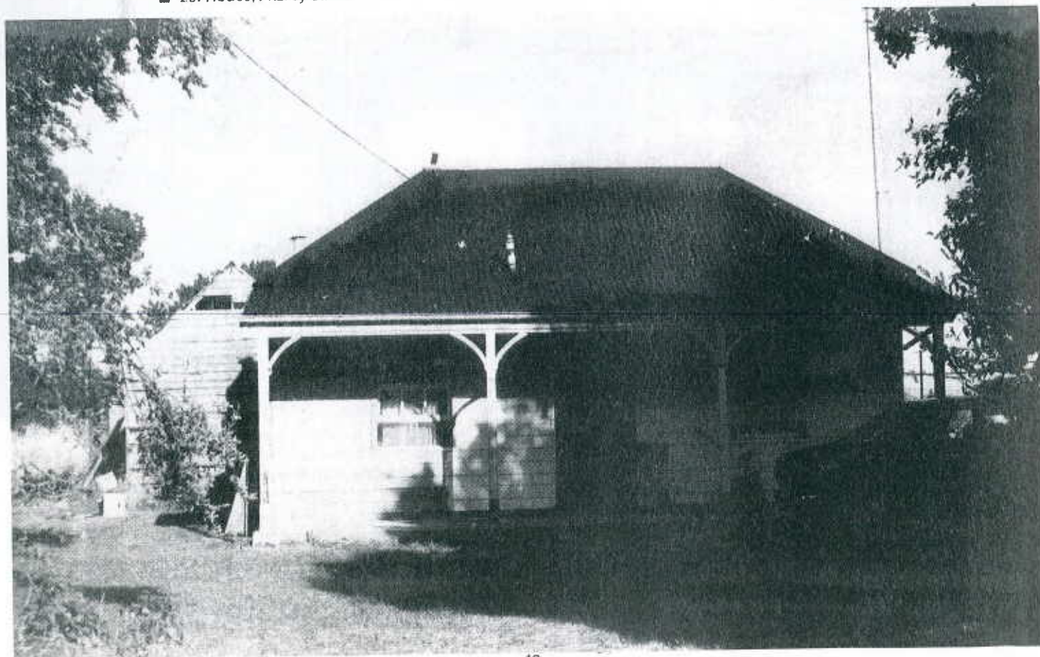
■ 29: House, Fitzroy Street
