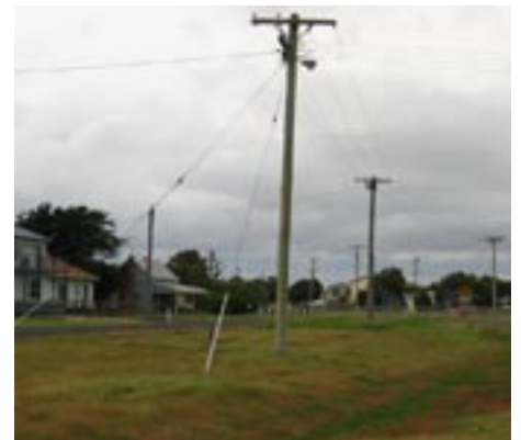
Typical housing and dominant powerlines
