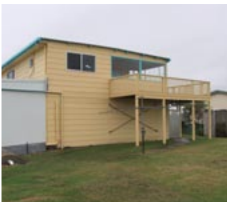
Substantial house on filled site
