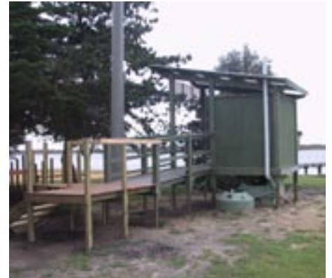
Foreshore composting toilet
