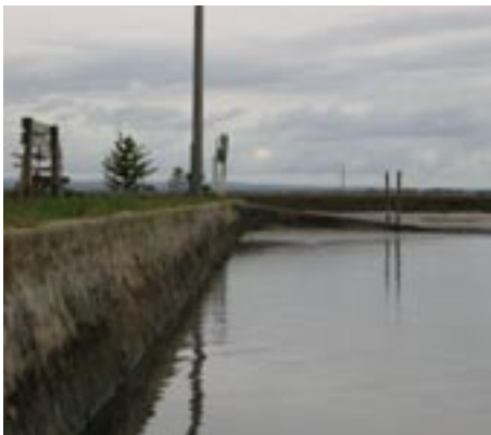
Boat launching ramp at Manns Beach
