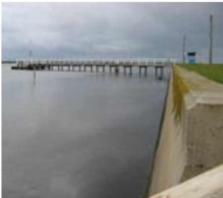
Manns Beach seawall and jetty
