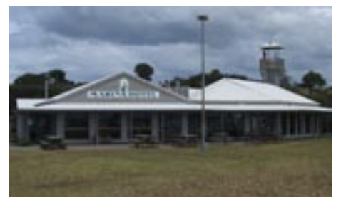
Commercial development at marina
