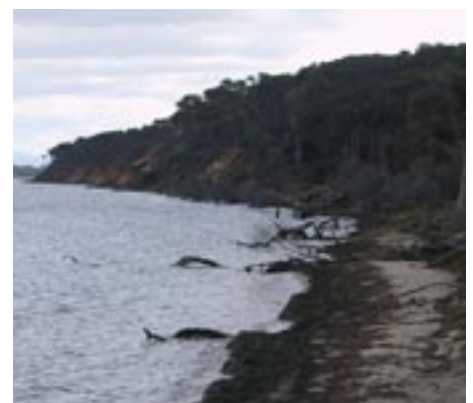
Erosion on Lake Victoria foreshore
