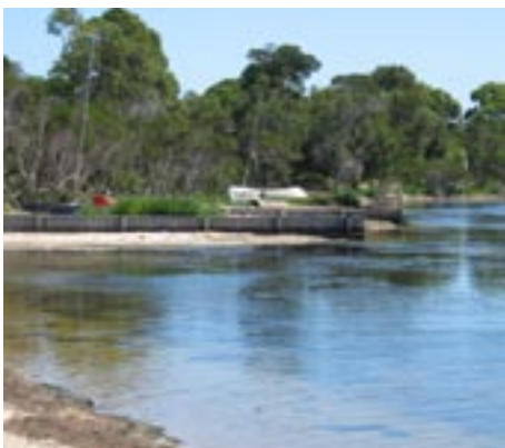
Groynes to control foreshore erosion
