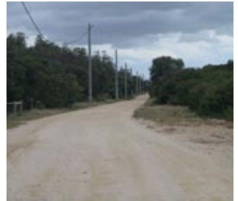
Unmade roads extend through most of the estates
