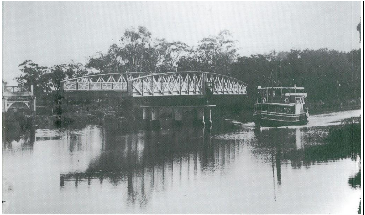
SWING BRIDGE OPEN TO ALLOW THE PASSAGE OF THE STEAMER S.S. DARGO
