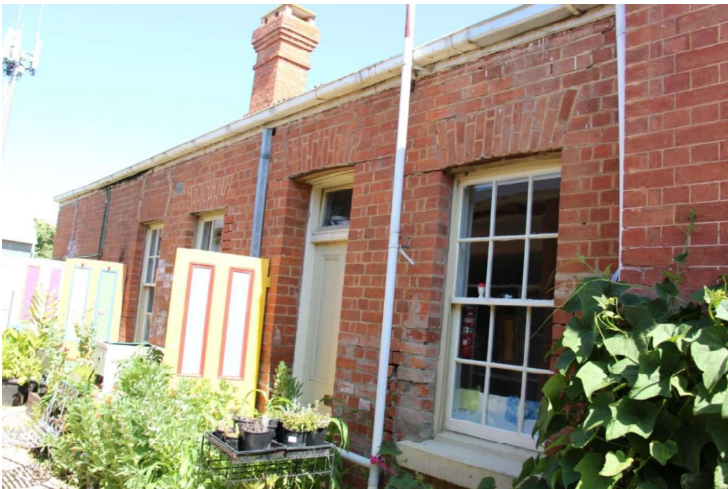
Figure D4. The north elevation of the council chambers, towards the rear, with its six-over-six timber windows.
