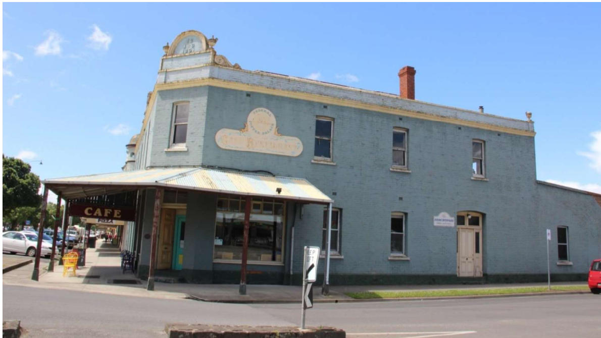
Figure D1. The two-storey building has a hipped roof clad with corrugated iron, and is constructed of handmade tuck pointed red-bricks (overpainted), with a brick plinth. Both main elevations have a rendered (overpainted) parapet above a bold cornice moulding; the southern elevation retains the urn at the end.
