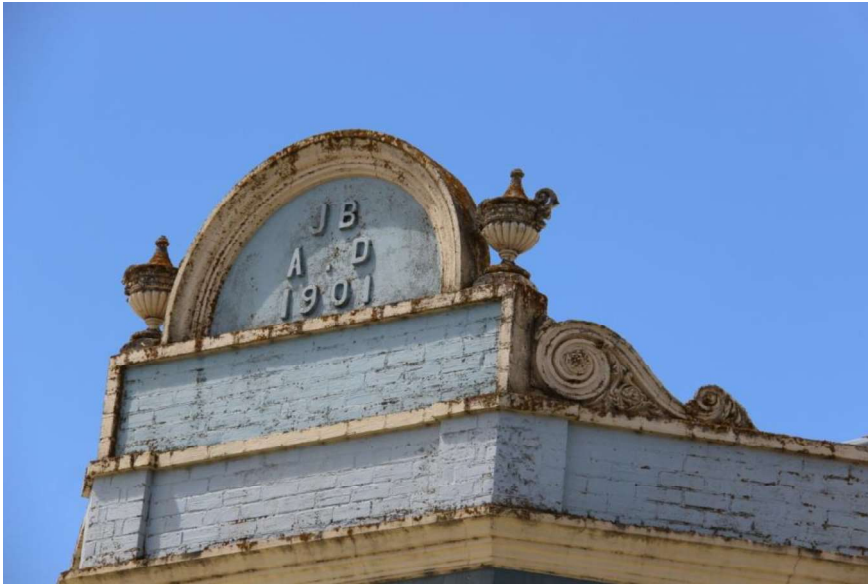
Figure D2. The chamfered corner entrance has a round-arched section above the parapet, with consoles and urns either side. The face of the arch bears the words 'JB A.D 1901' in relief.
