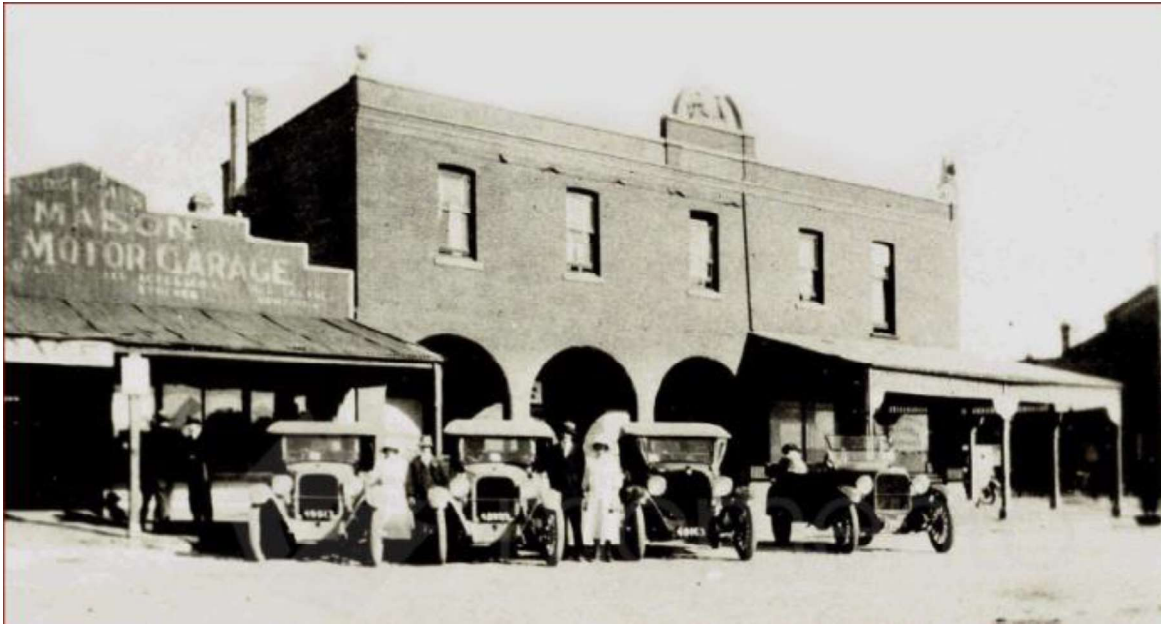
Figure H4. A photo taken after c1914 (when the Strand Hall was built to the south) The full extent of the west elevation was evident, with the return verandah to the shopfront (Stone n.d.:31).
