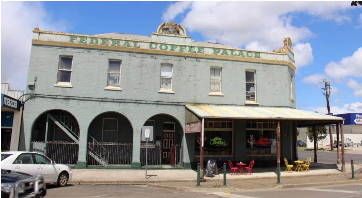
Figure D3. The west elevation comprises the 1901 section (with the verandah) and c1905 section (loggia with the round arches to the ground floor). Above the centre of the parapet is a projecting section that holds the coat of arms.
