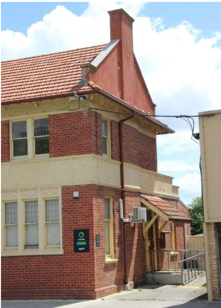
Figure D3. The north elevation with the domestic entrance porch and recently added concrete ramp for access.
