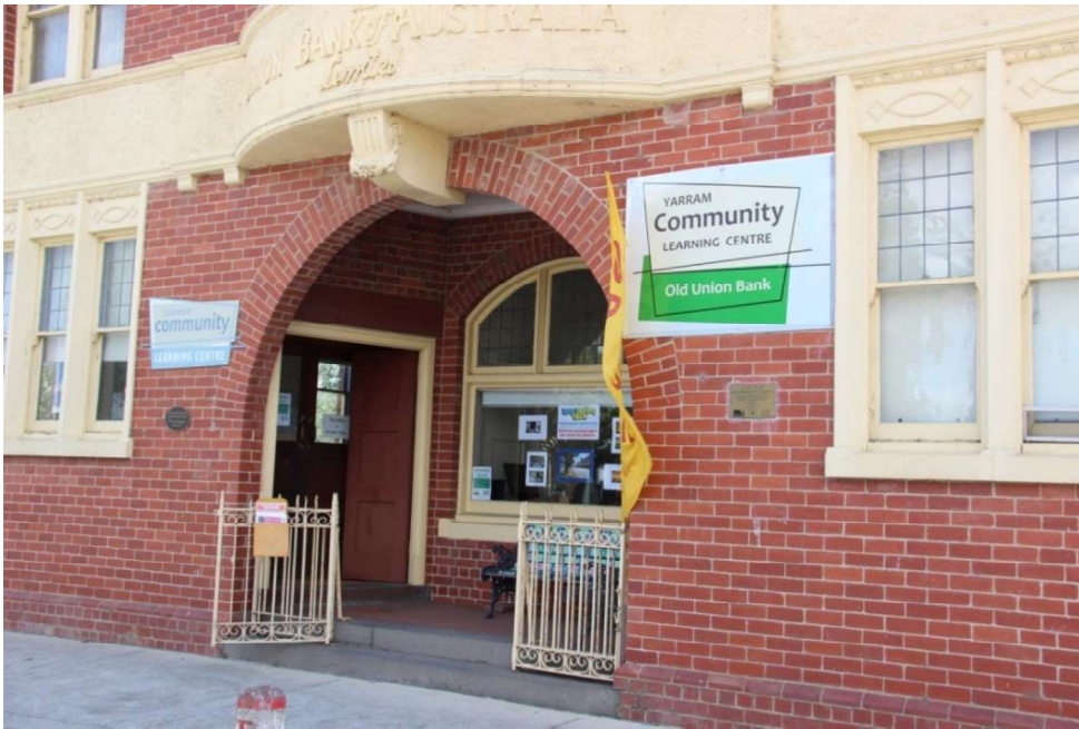
Figure D2. A detail of the entrance with its large semi-circular red brick arch and (c1950s) wrought-iron gates, in front of the large window with geometric leadlight, which is also evident in the other timber-framed windows.
