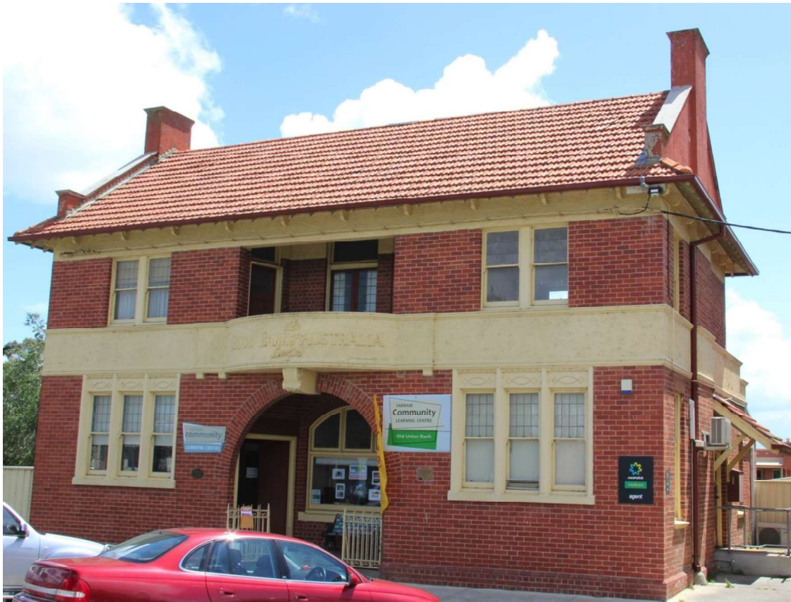
Figure D1. The facade of the bank with the predominantly gabled roof clad with terracotta tiles, exposed eaves, a pair of parapeted gable ends which have small hipped extensions for the continuation of the eaves and central semi-circular red brick arched entrance and wide bank of (over painted) render.
