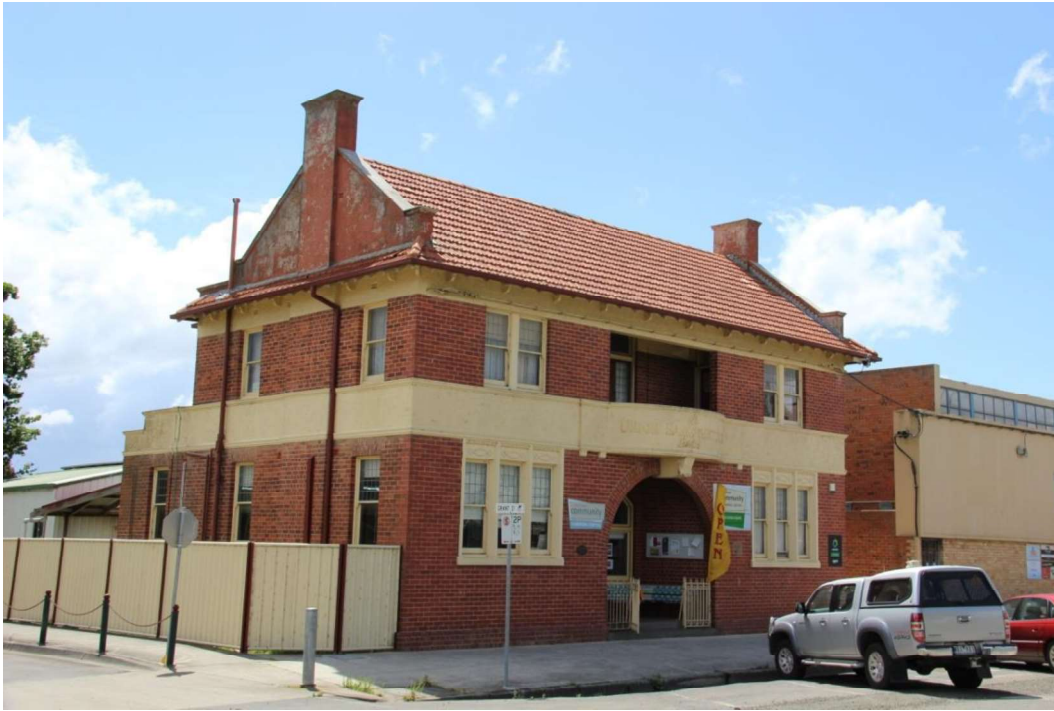
Figure D4. The facade and south elevation, showing the single-storey section to the rear and modern skillion verandah.
