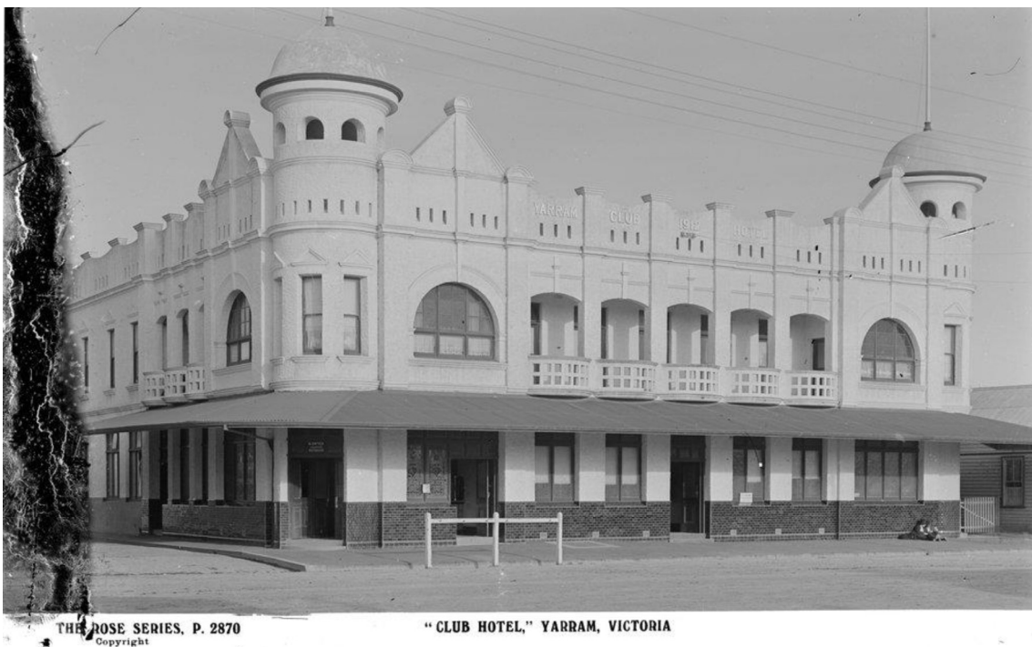
Figure H3. This photo dating between c1920 and c1954 showed the facade and north elevation of the Yarram Club Hotel in clear detail. The building above the verandah appeared as it does in 2015, although the colour application of light and dark is different. At ground level, there was an entrance at the north end (south of the corner entrance) that has since been closed, otherwise the openings were the same as those that remain in 2015 (SLV, H32492/4104).
