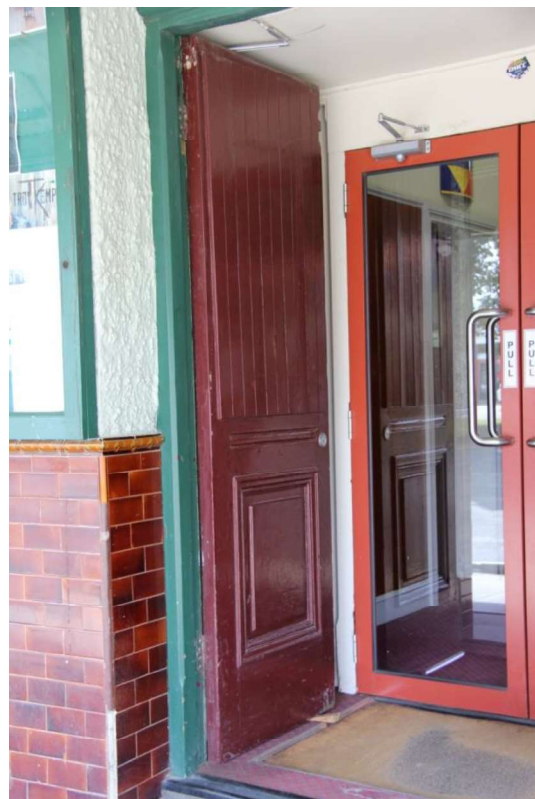
Figure D4. The southern entrance (left) at the base of the tower, and the central entrance to the facade (right). Both have the original timber panelled doors (that have had the top panel of glazing covered over).
