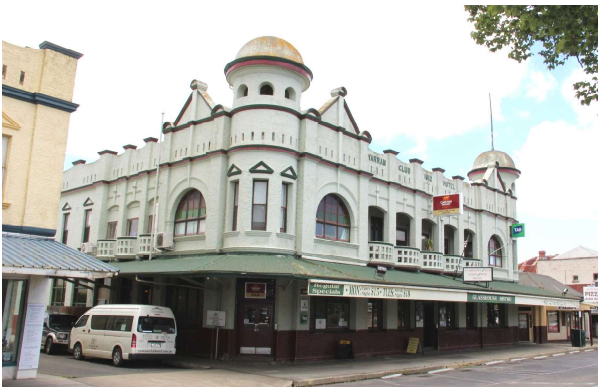
Figure D2. The form and detail to the facade is repeated on the side elevations, including the parapet and pediments, Diocletian windows and the balconies to openings.
