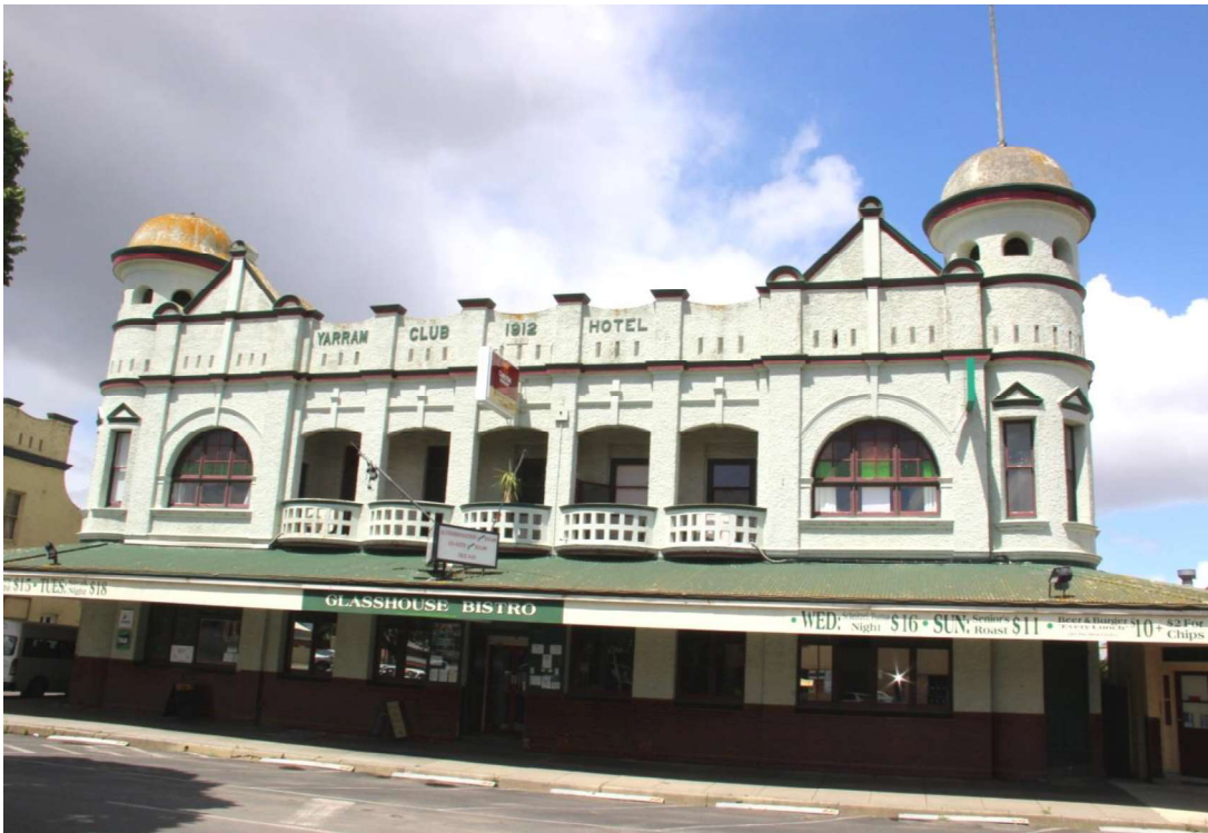
Figure D1. The substantial two-storey building has three main elaborate elevations with Classical details and prominent corner towers, and is highly visible throughout the town.
