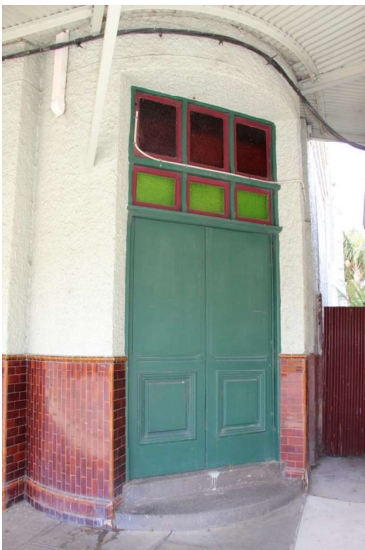
Figure D4. The southern entrance (left) at the base of the tower, and the central entrance to the facade (right). Both have the original timber panelled doors (that have had the top panel of glazing covered over).
