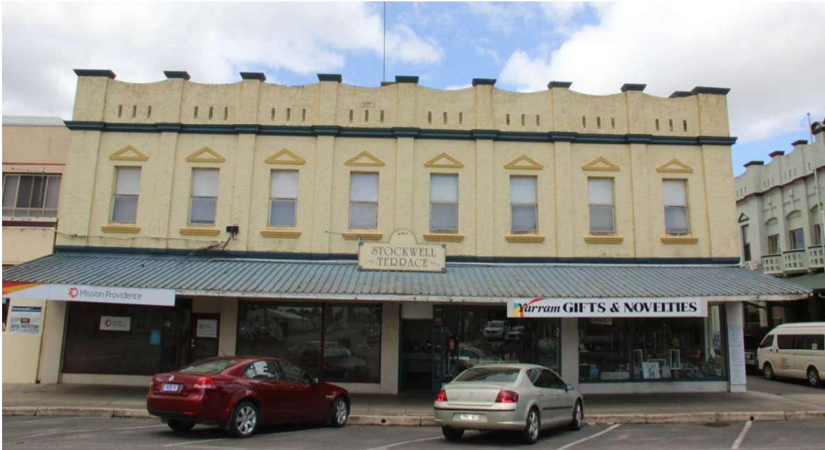
Figure D1. The symmetrical facade is dominated by the tall parapet, Classical details and very wide verandah to the ground floor. The first floor and parapet are divided into eight bays, created by engaged pilasters, which gives the building a strong vertical emphasis.
