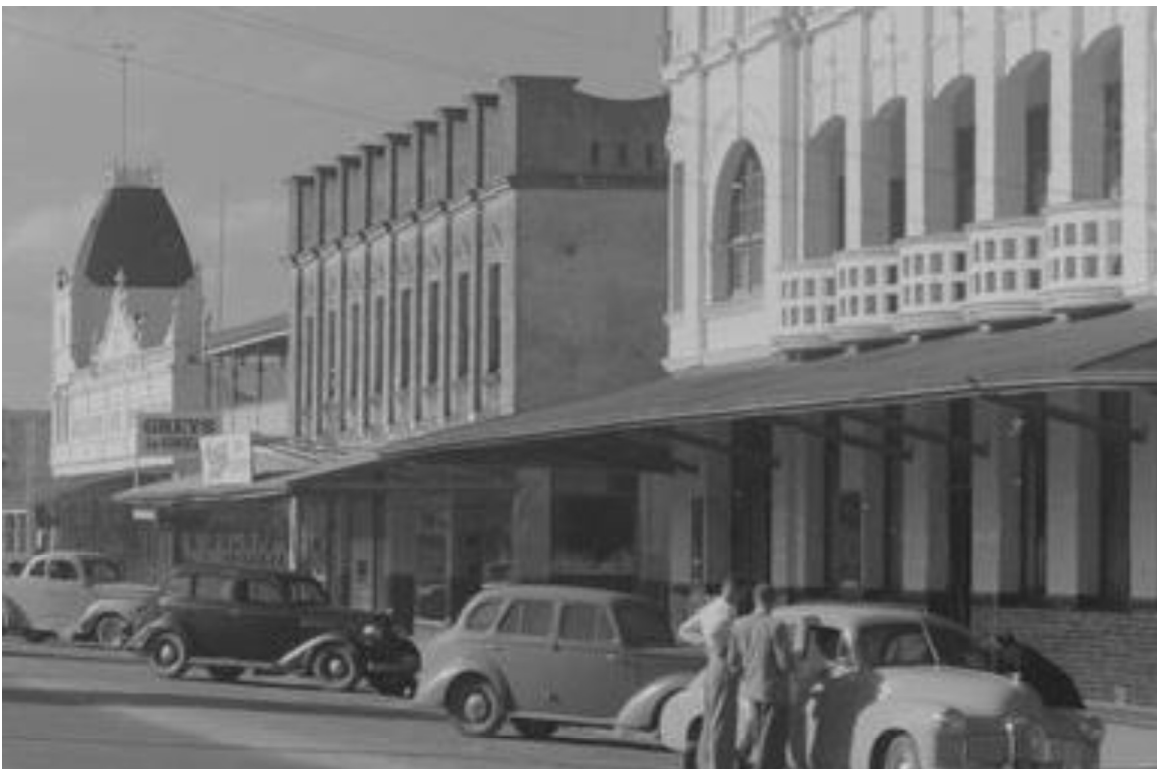
Figure H4. A photo dating between c1945 and 1954 also showed the Stockwell Building from the south, now painted, and in darker tones, with the parapet in a contrasting tone. The photo (as does Figure H3) showed that the original shop fronts had large panels of glazing between large piers, and the piers had a dark coloured dado, the same height as the one on the Yarram Club Hotel. (SLV H91.50/526).
