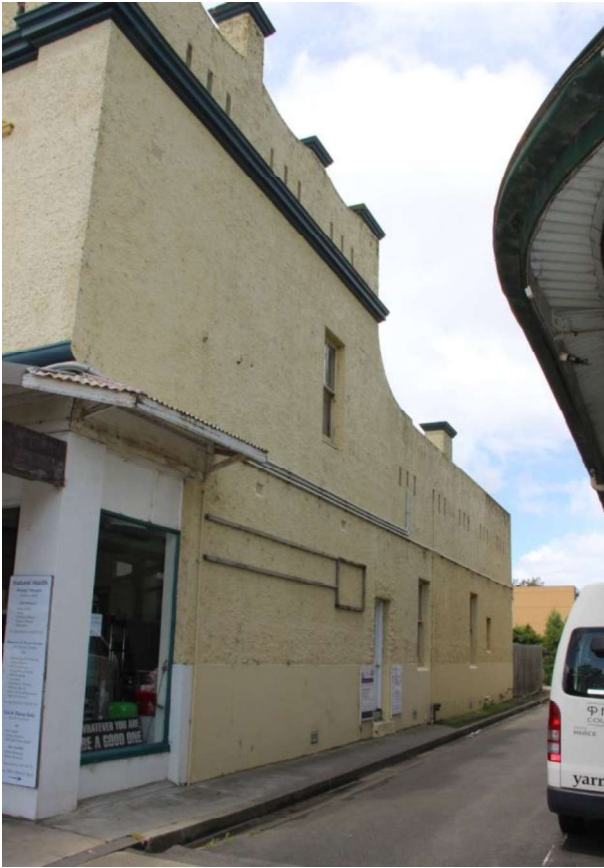
Figure D3. The south elevation. The parapet continues on the side elevations, reducing to single-storey height at the rear of the building. At ground level is a dado of smooth render which was originally a darker colour than the rest of the building. A small shopfront window is located on the south elevation, as appears in the historic photos
