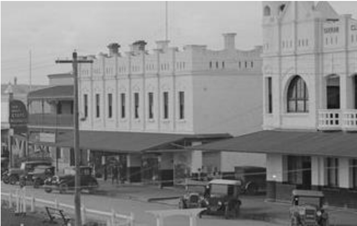
Figure H3. A photo dating to c1930 (by the date of the cars), shows the Coffee Palace was predominantly a single light colour like the Yarram Club (which may have been the original colour of the render without paint) except for the smooth render dado along the ground floor level and side wall (SLV: H32492/5527).
