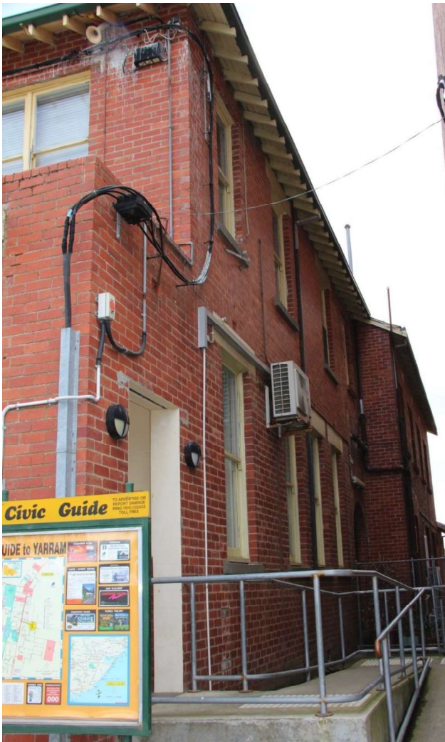
Figure D3. The north elevation. The 1913 section of the first-floor has the wide eaves and exposed rafter ends. To the rear of this is the 1950s first-floor addition, built on top of the 1913 single-storey residence.
