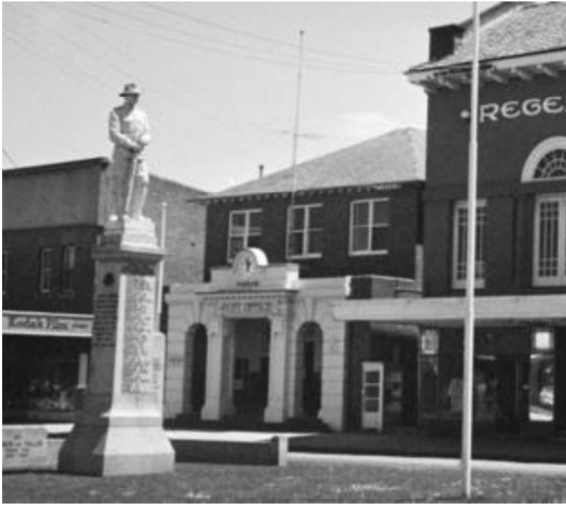
Figure H4. The post office in c1969. The first floor balcony had been in-filled by this date. The clock and name had been installed on the entrance porch (SLV).
