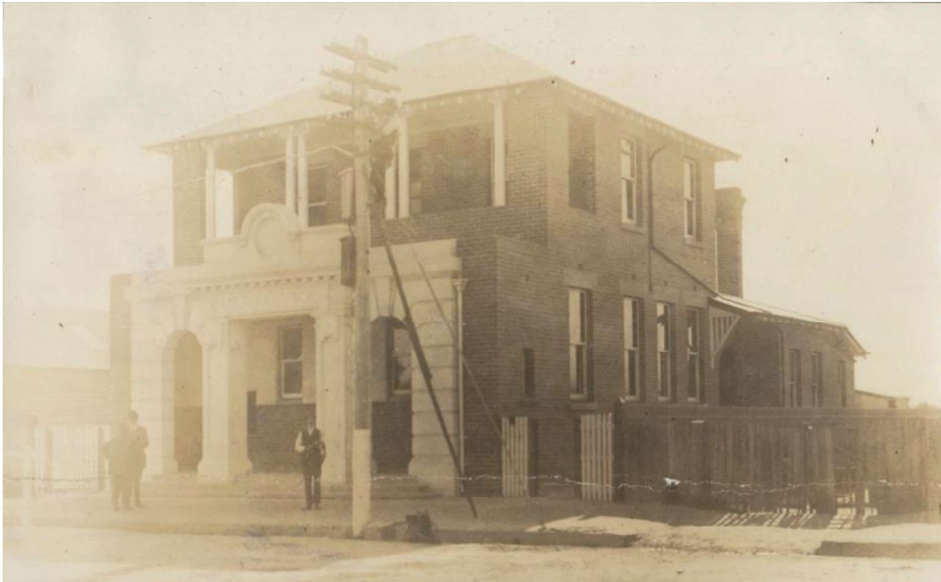
Figure H1. Photo of the post office dating between 1917-1930. The clock had not been installed and the first floor retained its recessed balcony supported on elegant classical columns. The single storey residential residence is visible on the side elevation (SLV).
