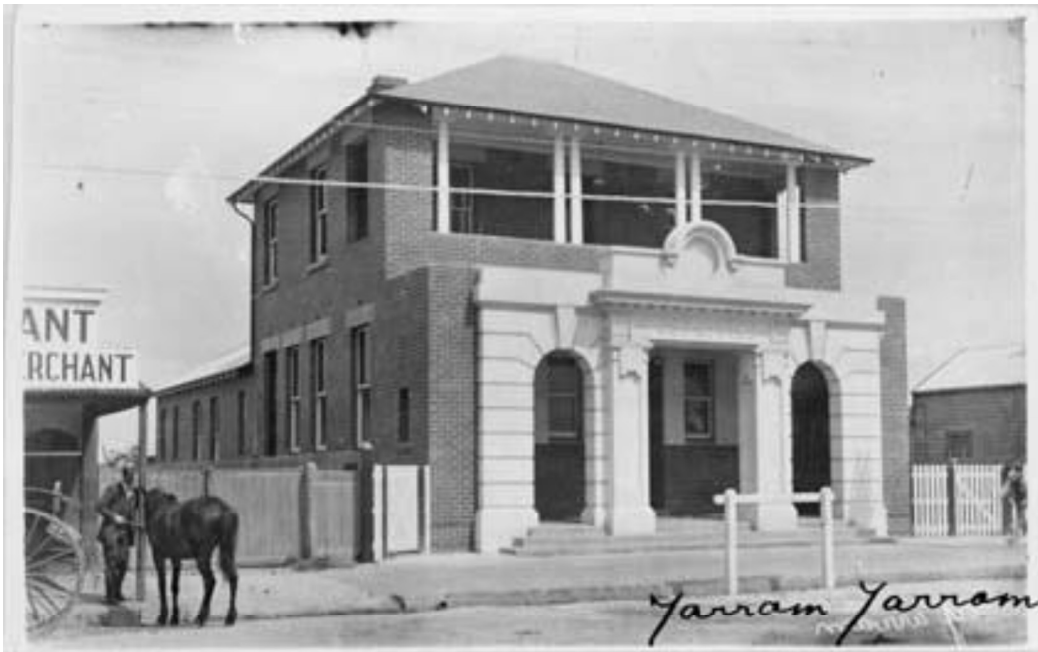
Figure H2. The post office between 1917-1930 in its original unpainted state. The first floor was only three rooms deep (later extended) (NAA).
