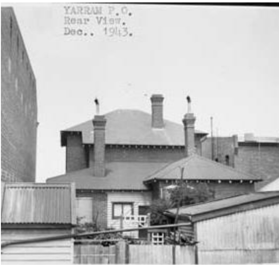
Figure H3. The original rear elevation of the post office in 1943, prior to the extension of the first-floor in the 1950s (NAA).
