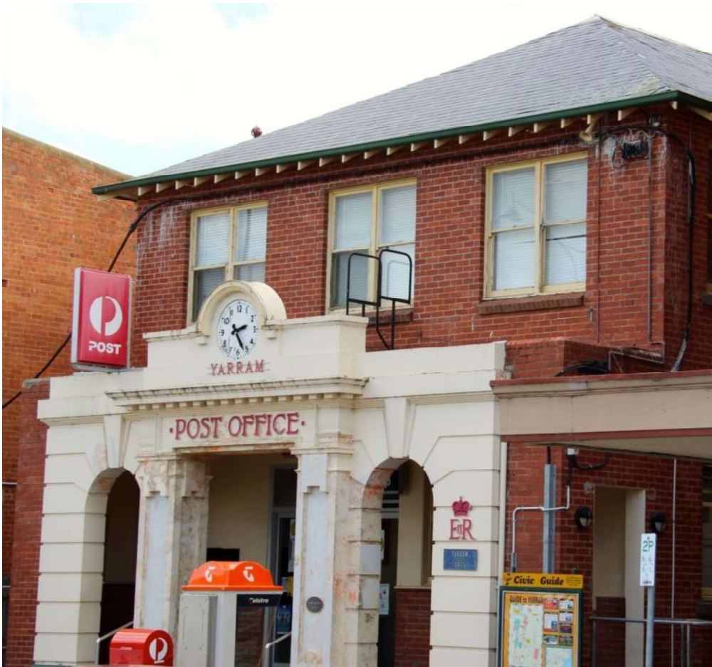
Figure D1. The post office with its hipped roof clad with slate and wide eaves with exposed rafter ends, and the rendered Palladian-inspired Classical portico dominating the facade. The first floor balcony was in-filled with windows by c1969.
