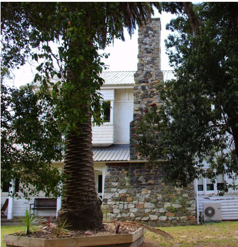
Figure D4. The palm trunk, and Arts and Crafts unpainted chimney seen from King Street, on the southern boundary of the property.
