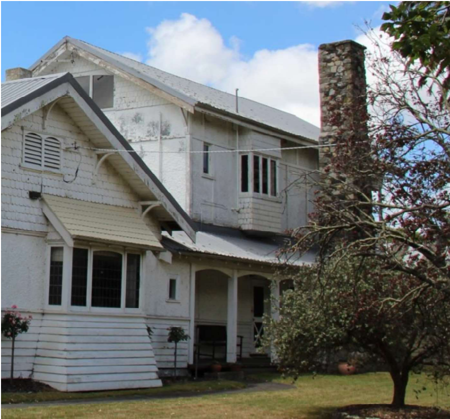
Figure D3. The 1920 section of the house is two-storey and similar in design to the original 1912 section. It is notable for its large two-storey external stone chimney.
