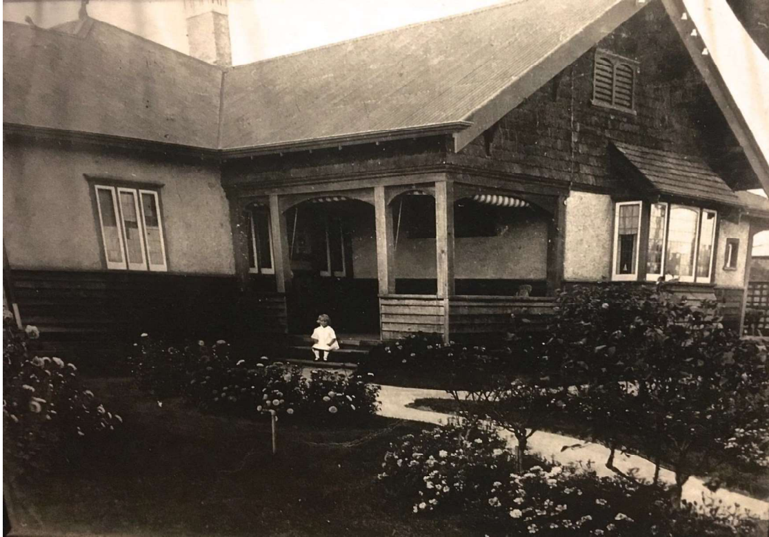
Figure H1. The original single-storey section of the house (Fisher 2016).
