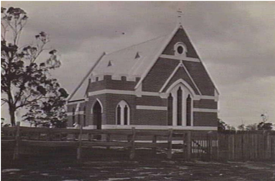
Figure H1. An early photo dating between 1895 and c1909 showed the facade and north elevation of the church. The nave of the church appeared as it does in 2015, however, the spire had not yet been constructed on the tower base. The new render is still a light grey colour (SLV, image no. b23150).
