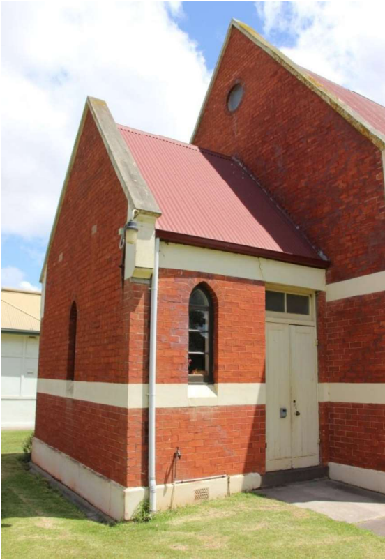
Figure D4. The gabled-end of the rear (east) elevation of the church has a round opening, above a chancel with a rendered parapeted gable. Timber doors with a highlight provide access off the north elevation. Small pointed-arch windows with three-paned casement windows (with clear glass) appear on each side.
