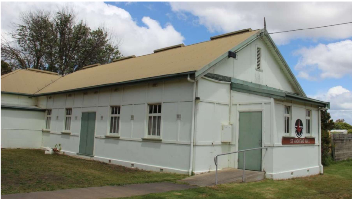
Figure D5. To the south of the church is the 1929 hall which underwent extensions in 1955, which comprised the hipped section to the rear with one-over-one sash windows. Both sections of the hall have a rendered plinth and are constructed of rendered brick to the bottom third of the wall, which is incised with ruled lines to create an ashlar effect. The top 2/3 of the wall and gabled-ends are clad with fibro-cement sheets and strapping (all overpainted).
