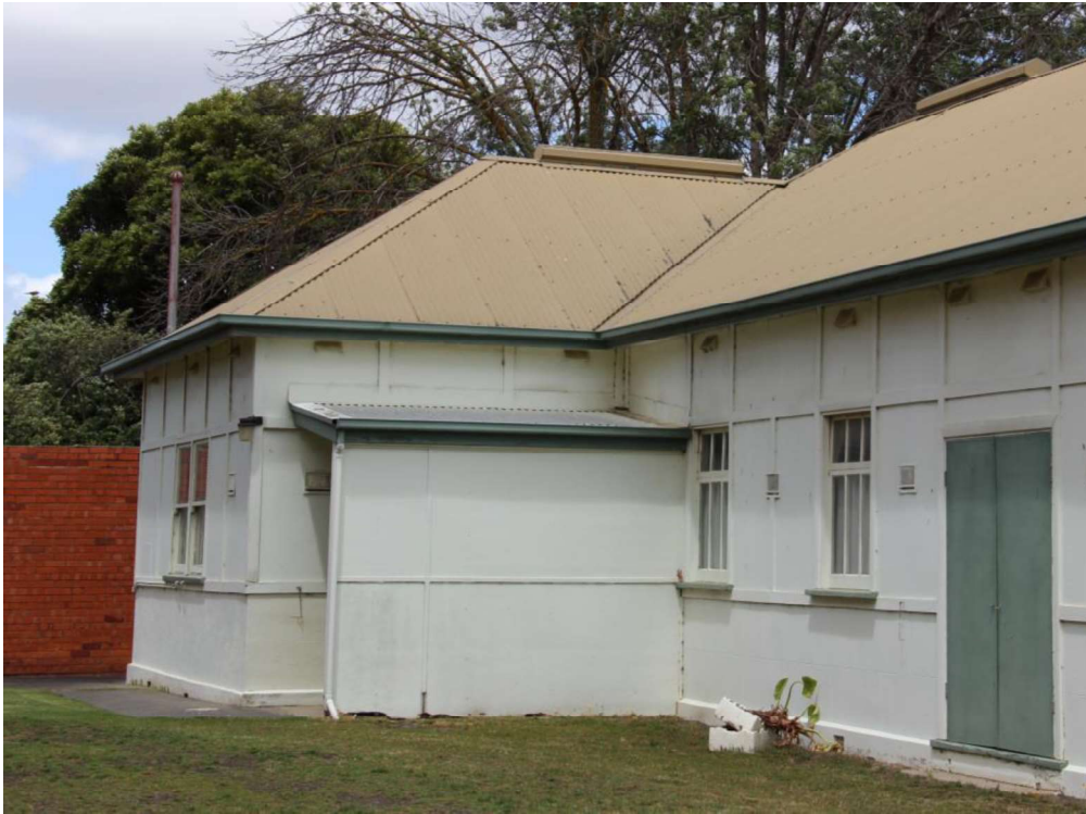
Figure D6. The 1955 hipped-roof addition to the rear imitates the architectural details of the 1929 section, but has one-over-one sash windows. A small skillion-roof section is enclosed with one wall, located on the west side of the 1955 section.
