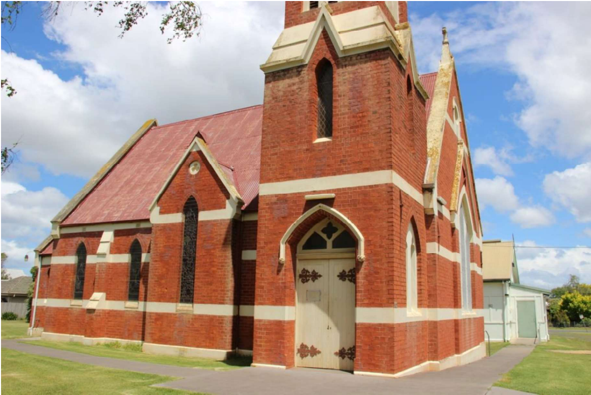
Figure D2. The north elevation contains the entrance on the north side of the tower. The pointed-arch opening has a label moulding stopped by rosettes, and recessed entrance with double timber ledged and framed doors (with ornate metal hinges) and a highlight with a quatrefoil motif.
