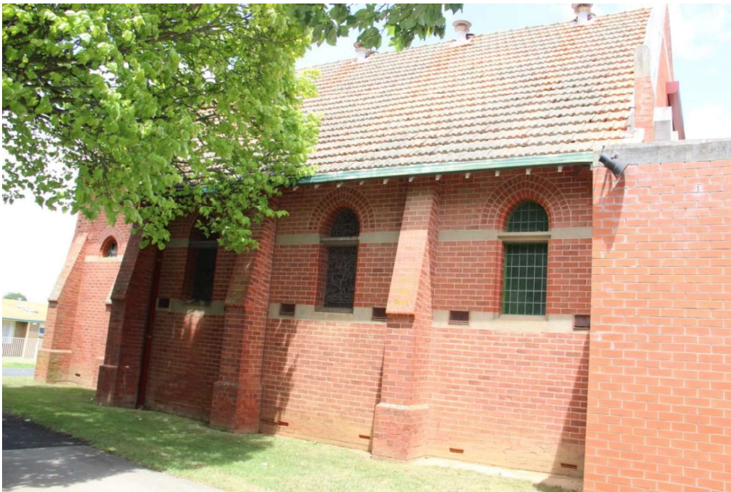
Figure D2. The north elevation. The side elevations are broken into bays by wide brick buttresses. The bays have a single (slightly pointed) arched window with three rows of bricks voussoirs radiating above. Two bands of decorative render run across the wall planes of the side elevations at sill level and the spring point below the arch.
