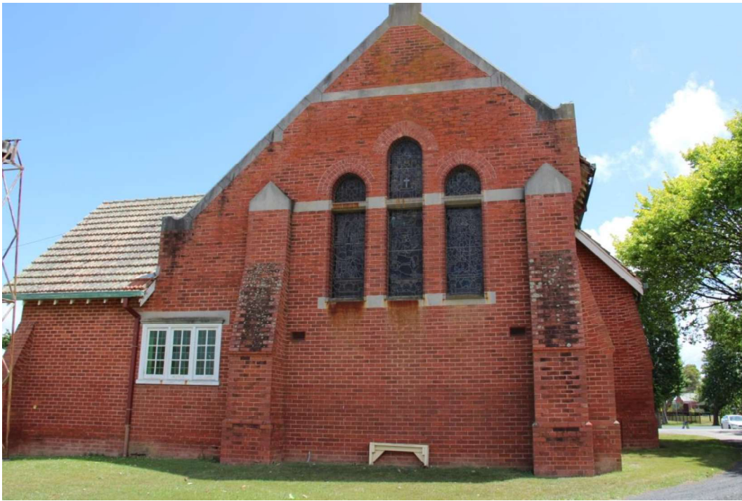
Figure D3. The rear (east) elevation has the same detail as the facade and three large (slightly pointed) arch windows with stained glass. To the left of the rear elevation is the wall of the south porch and a grouping of three square-headed windows.
