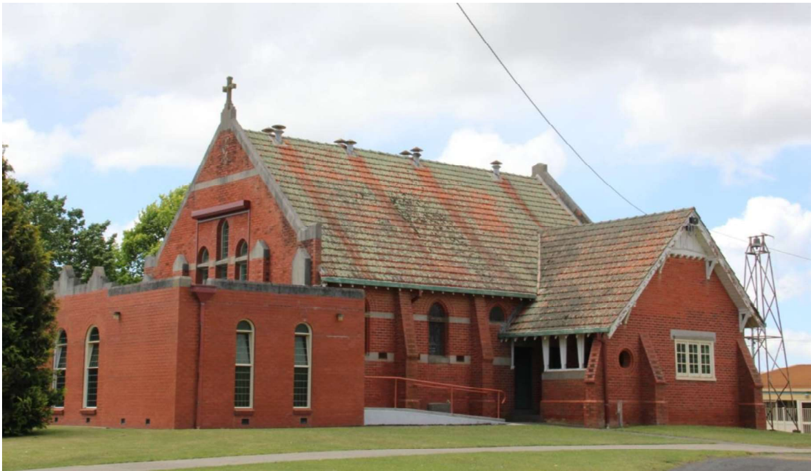
Figure D1. The church is constructed of tuck pointed red brick, with a tall brick plinth, a steeply-pitched roof clad in terracotta tiles (with lichen) and rendered parapeted gables. Round metal vents are located along the ridge of the roof. At the rear of the southern elevation is a large gabled-roof porch, built in 1918. A modern single-storey flat-roofed narthex has been added to the facade of the building.
