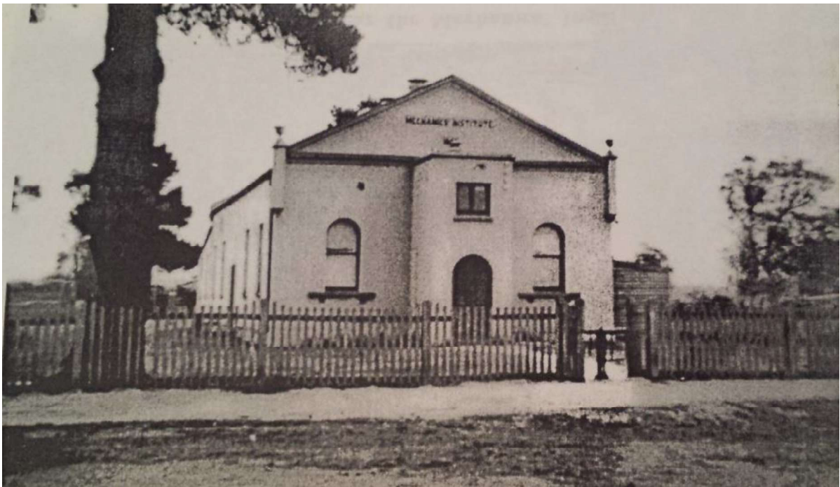
Figure H1. An early photo (exact date not known) of the hall with its entrance porch on the facade, (Note the porch appears to have been altered at the top, to accommodate a biobox for movies, but the whole structure was removed, filled in, and a new entry placed on the south-east elevation in 1973) (YDHS heritage trail).
