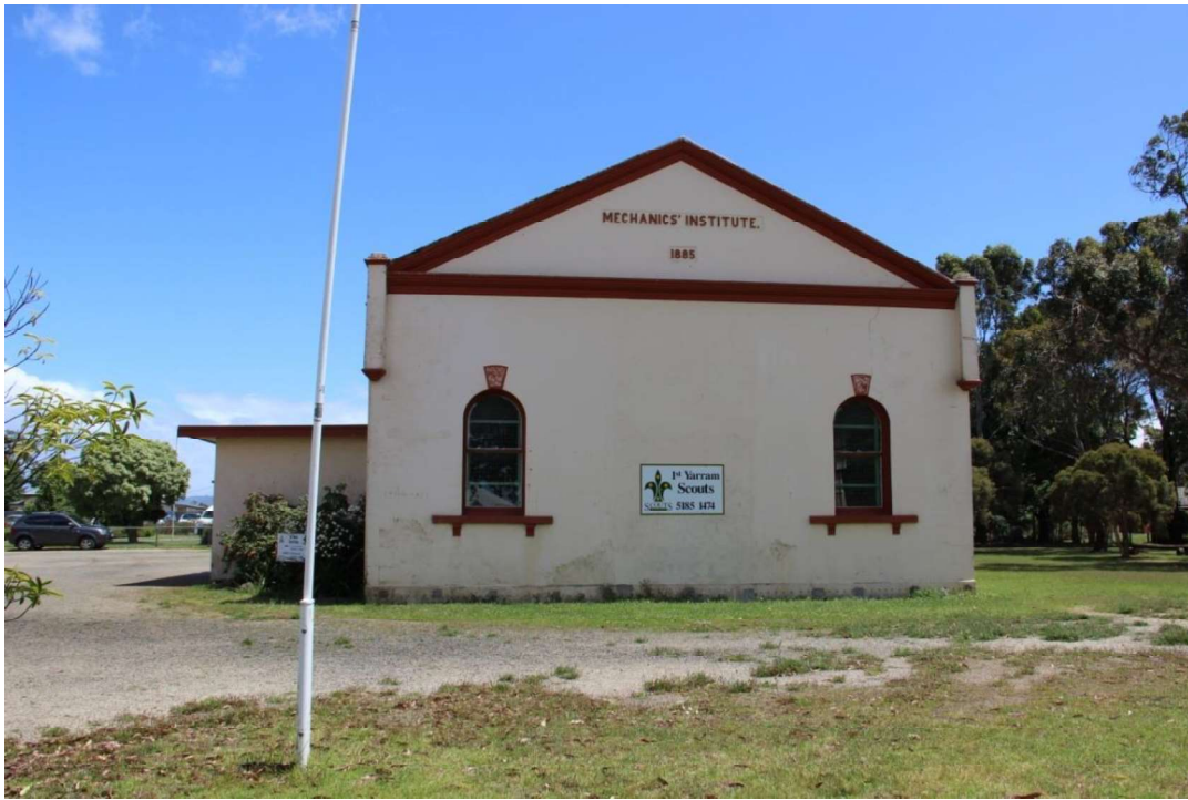
Figure D1. The facade of the hall which faces the South Gippsland Highway. The bold parapeted gabled-end is framed by a bold moulding, creating a pediment effect. The original front door and porch have been removed.
