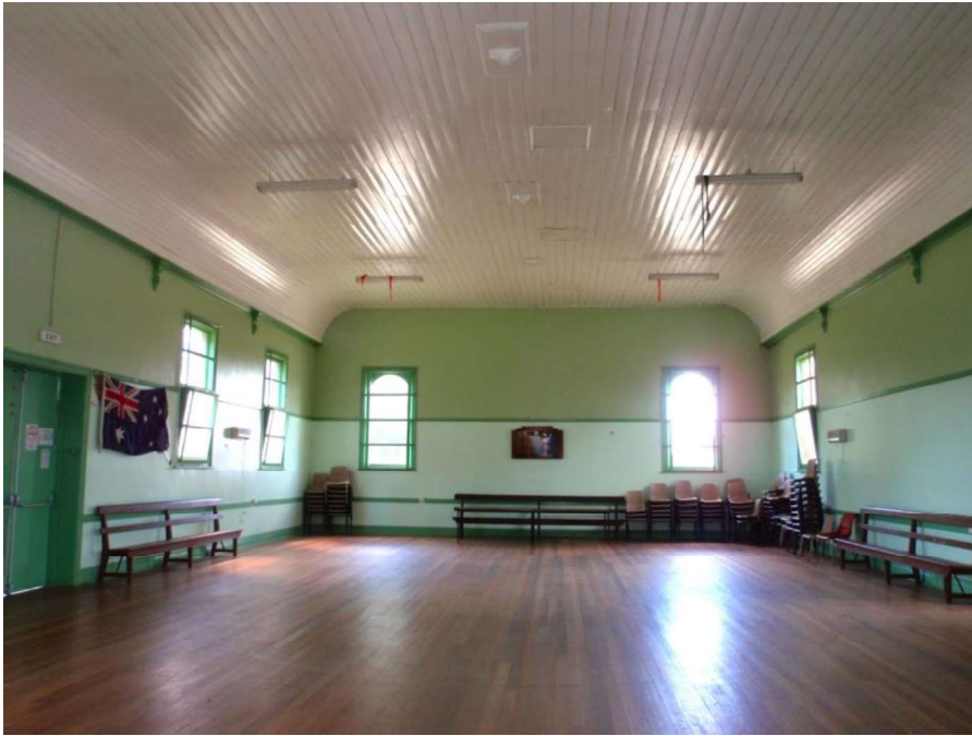
Figure D5. View of the interior looking towards Church Street (where the front entry door has been blocked up). Note the timber panelled coved ceiling, picture rail moulding and classical consoles.
