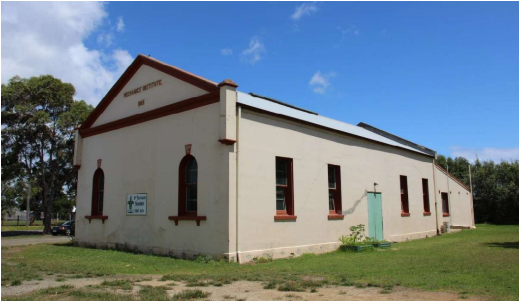
Figure D3. The north-east elevation has four timber windows and a central entrance.
