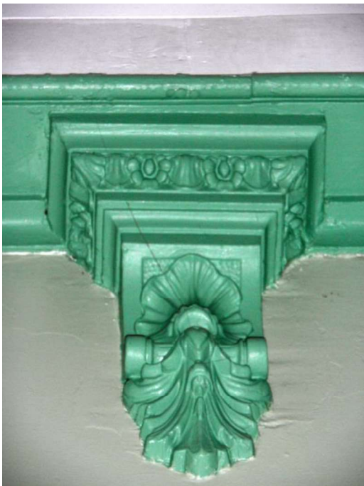
Figure D6. Detail of console decoration inside.
