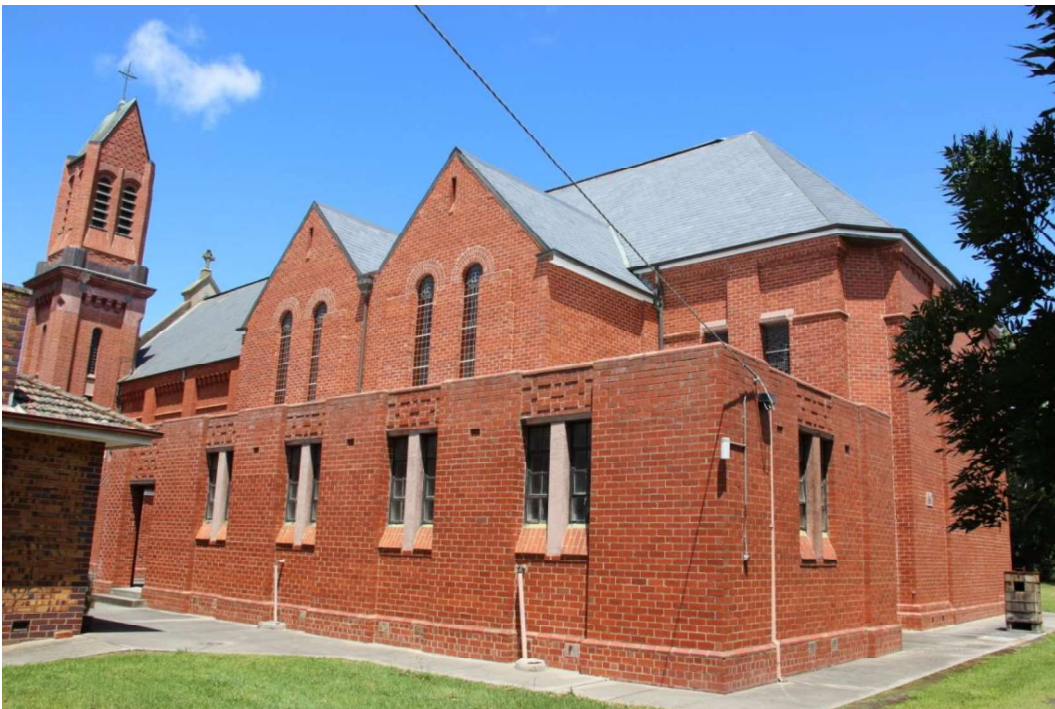
Figure D3. The north elevation. To the rear of the 1915 church, at the west end, is very large brick addition constructed in the 1960s. This later addition is identifiable by the later brickwork and single-tiered brick plinth. The 1960s addition comprises the tall double-gabled transepts, the chancel end, and the flat-roofed addition off the north elevation.
