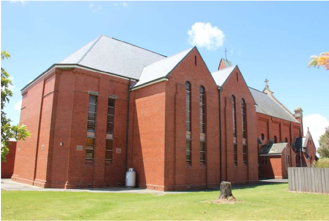
Figure D4. The two smaller gabled-roof rooms projecting off the centre of the side elevations were also constructed in the early 1960s.
