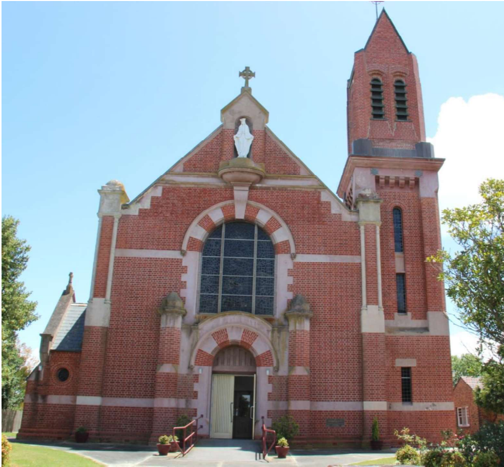
Figure D1. St Mary's Catholic Church is a very large church constructed of tuckpointed red brick, with a two-tiered plinth to the original 1915 building. A dominant element of the facade is the two semi-circular arches. To the right of the facade is a large square tower, with narrow openings to each face. The spire (above the bold cornice moulding) was constructed in the early 1960s.
