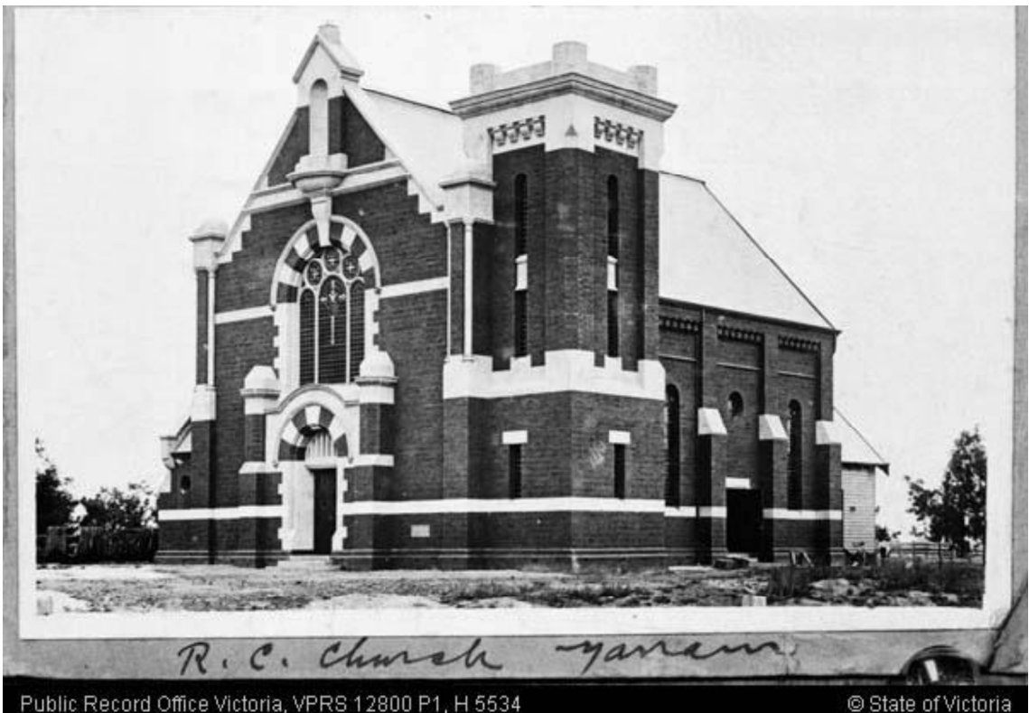
Figure H3. A second early photo (c1916). The original stained glass arrangement in the large window was evident (since replaced). The statue of the Virgin Mary has not been placed in the niche. The nave consisted of five bays, with a timber addition constructed at the apse end (PROV VPRS 12800 P1 H 5534).
