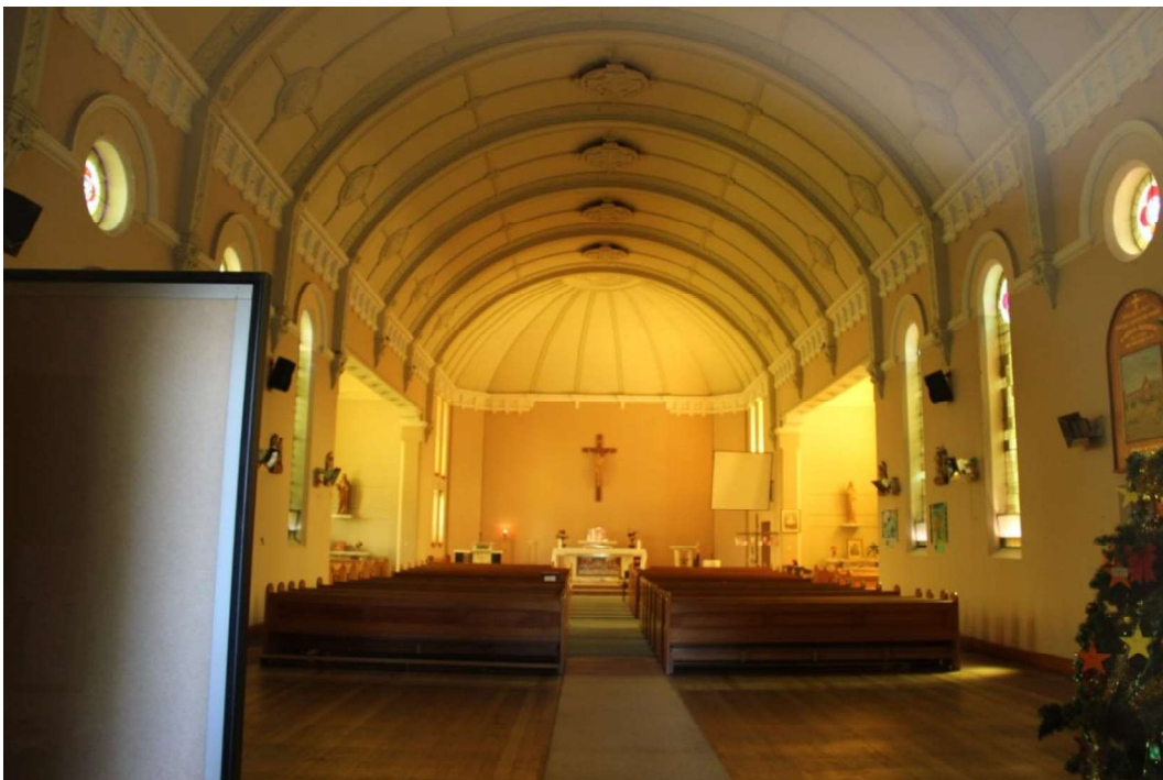
Figure D5. The interior of the church has a large barrel-vaulted ceiling lined in plaster. The 1915 extent of the church extends to the round-arched windows. The interior space and historic finishes of the interior are imbued with the rituals and aesthetics associated with worship, marriages, christenings, confirmation, and funerals.
