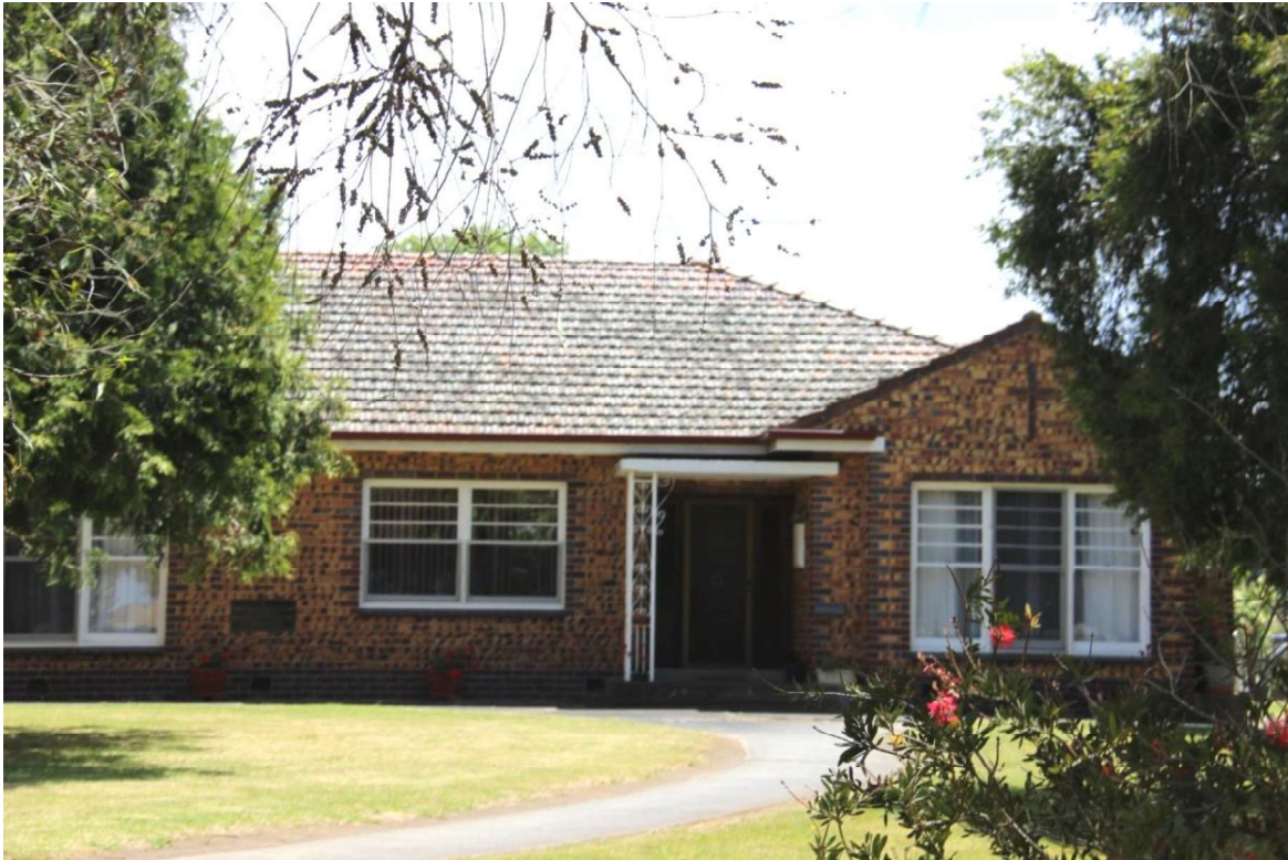
Figure D6. The large presbytery is constructed of tapestry bricks with dark brick quoining to the corners and openings, and a dark brick plinth. The shallow-pitched hip-and-gabled roof is clad with terracotta tiles. The house has groups of windows with a horizontal emphasis, each with horizontal glazing bars to the top sashes.
