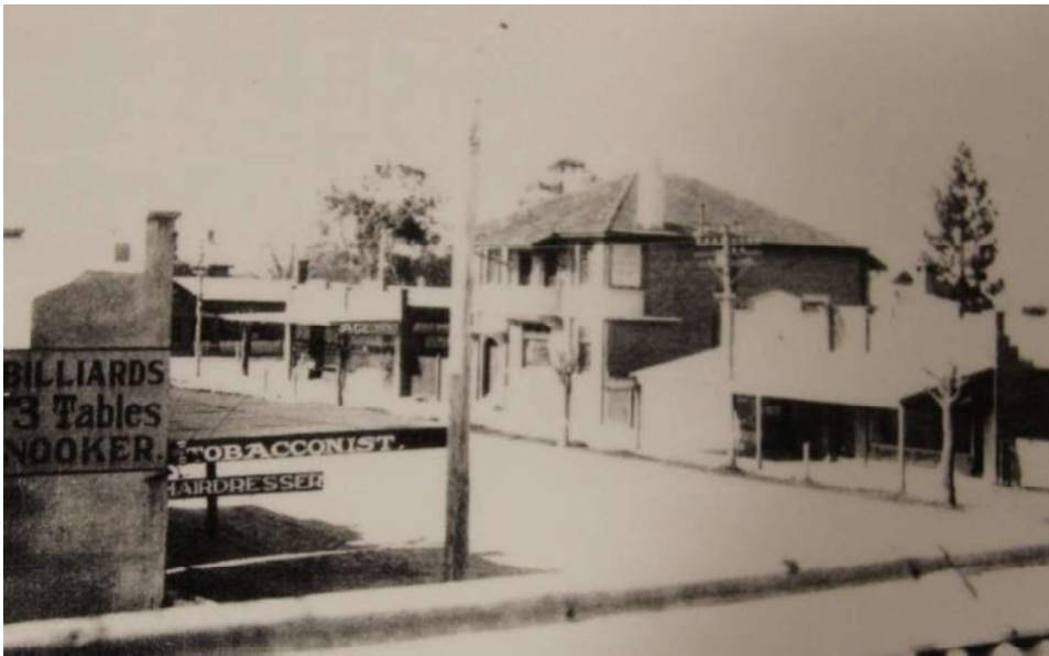
Figure H1. An early photo (date not known) (SDHS).
