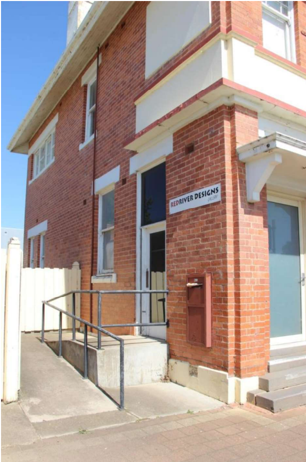
Figure D3. The north elevation with the altered entrance door, original bluestone steps, and single and grouped windows with rendered lintels and sills.
