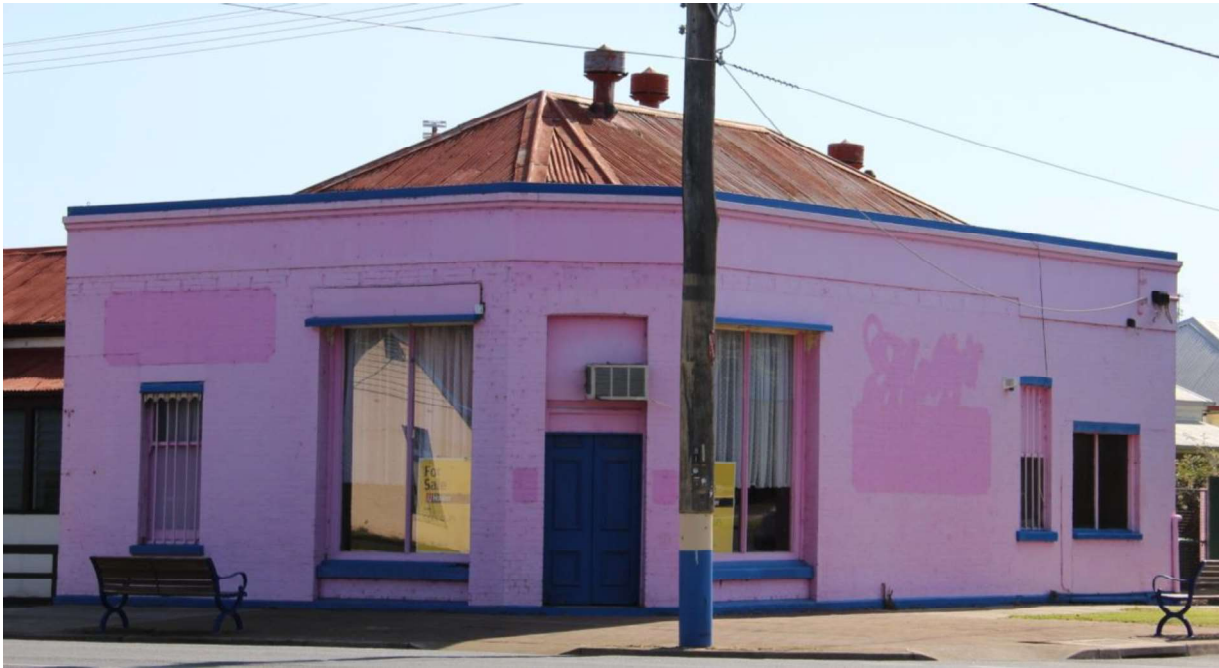
Figure D1. The large shop has a hipped roof clad with galvanized corrugated iron (overpainted) and a number of recent round metal vents to the roof. The shop is constructed of handmade red-brick (all overpainted) with a small brick plinth. The main elevations of the brick shop front Tyers and Blackburn Street, with a chamfered corner entrance and rendered parapet.
