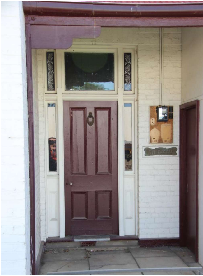
Figure D3. The Victorian entrance has a timber panelled door with sidelights above timber panels, and highlights with stained glass; above are radiating brick voussoirs. The bricks have been painted.
