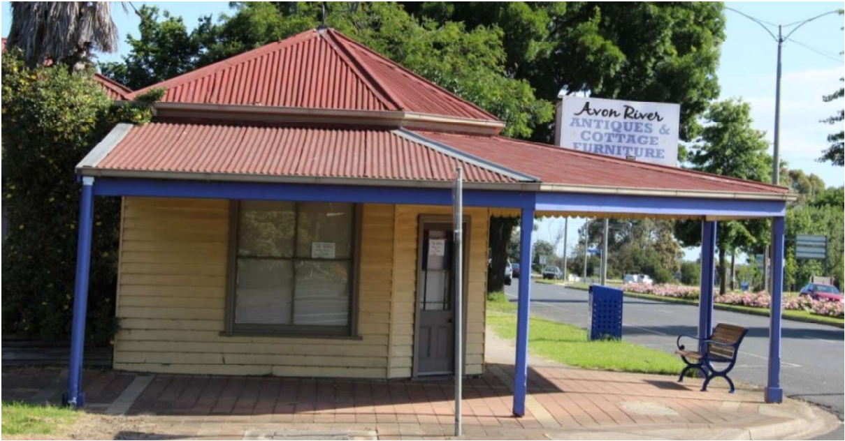
Figure D3. The small weatherboard corner shop has a faceted hipped roof clad in galvanized corrugated iron (painted). The original wide verandah extends over the pedestrian footpath, is clad with galvanized corrugated iron, has round-edged palings to the sides, and is supported by shop-chamfered timber posts, some with a timber base.
