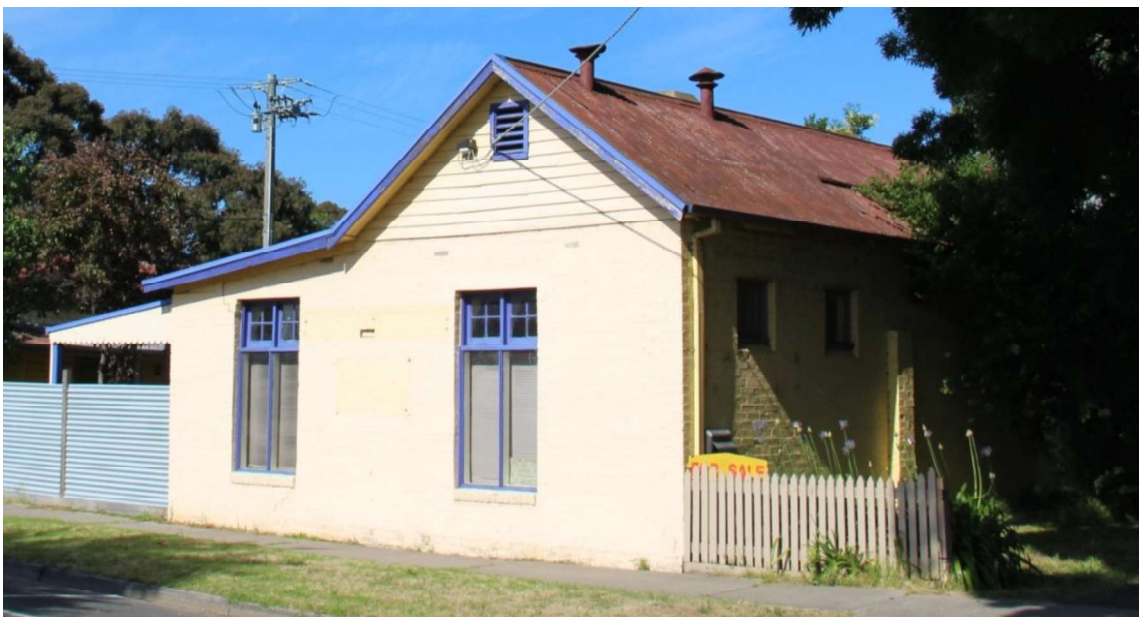
Figure D6. The east end of the bakery and to the right is the south elevation. The east elevation has two pairs of tall timber windows with a four-paned window to the top quarter, with brick sills and rendered (overpainted) lintels. These windows may date from c1900, but it is unlikely that they were located on this wall whilst the building was being used as a bakery. They may be second hand windows inserted into this wall when the building ceased being used as a bakery. The south elevation has small windows (one retains a four-paned window), also with brick sills and rendered lintels.
