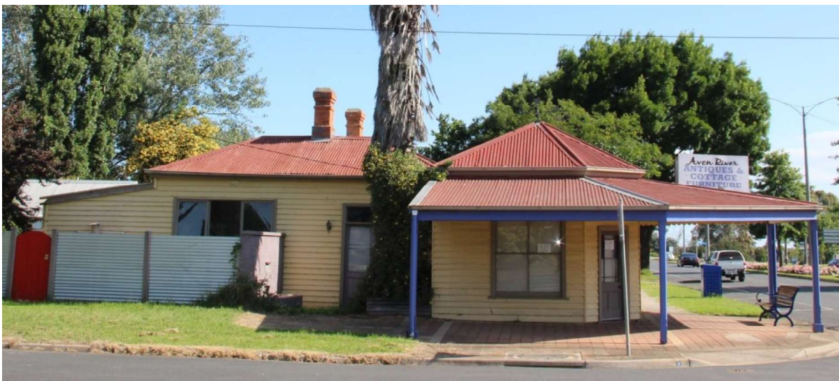
Figure D2. The north elevation has weatherboard cladding and modern timber doors and windows. The weatherboards continue to create a skillion-roof section at the rear (east) of the house.
