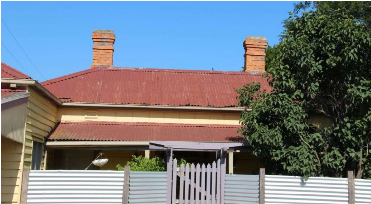
Figure D1. The house has an M-hip roof, clad with corrugated iron, and a verandah to the facade which returns on the south elevation. The house retains two corbelled brick (unpainted) chimneys that are constructed of handmade red bricks. A skillion-roof verandah is clad with corrugated iron (painted), supported by stop-chamfered timber posts.
