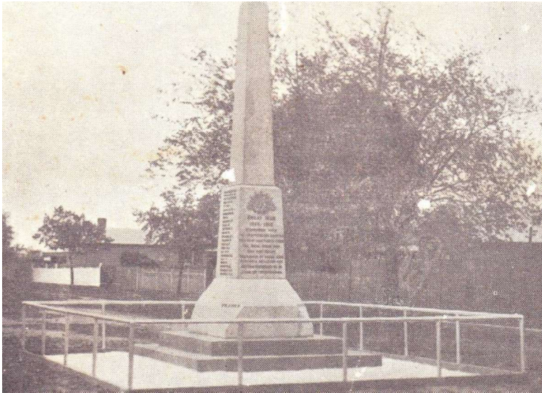
Figure H2. Early photo dating to the unveiling on 2 Nov 1924, of the Stratford Fallen Soldiers Memorial. Note the fence without a gate for access to lay wreaths. Also note the level of the ground (crushed white gravel?) hides the foundation concrete, which was incorrectly exposed in recent works (SDHS, ID No. 04003-28VSFH).
