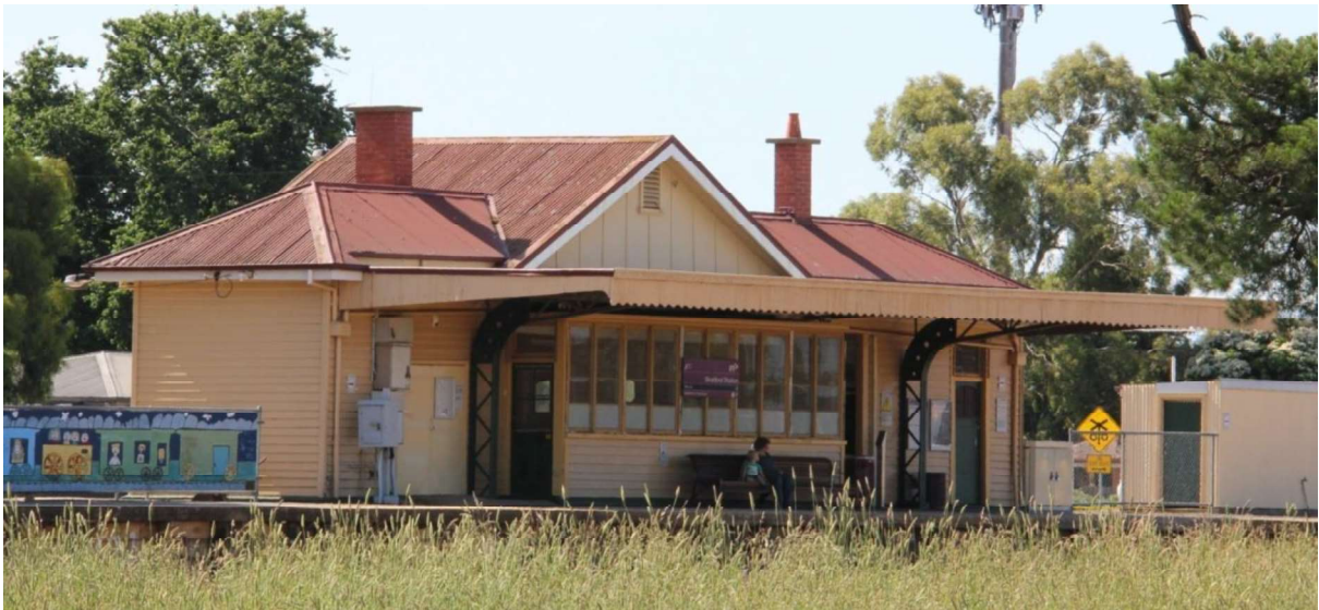
Figure D3. The platform (east elevation) of the station with its large metal trusses supporting the cantilevered awning with fluted and scalloped metal valances.
