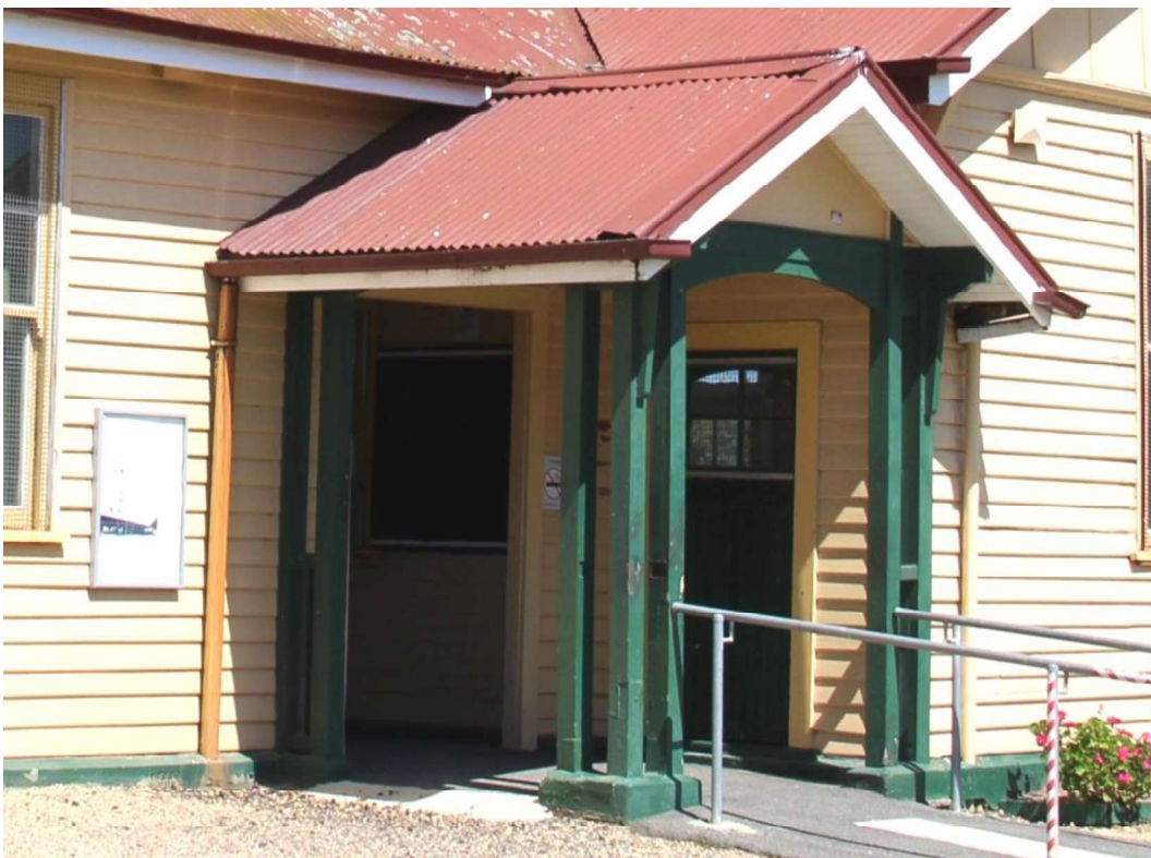
Figure D2. The gabled-roof entrance porch supported by pairs and triples of timber posts, with timber brackets and arch.
