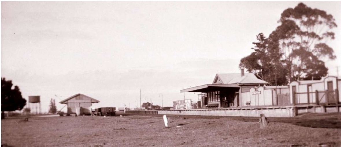
Figure H1A. An early photo (may date to c1930s-50s) of the station from the north, with the passenger platform on the right with a number of outbuildings lining the platform. On the left is a goods platform and corrugated iron goods shed, and the crane and water tower at a southern location (SDHS).
