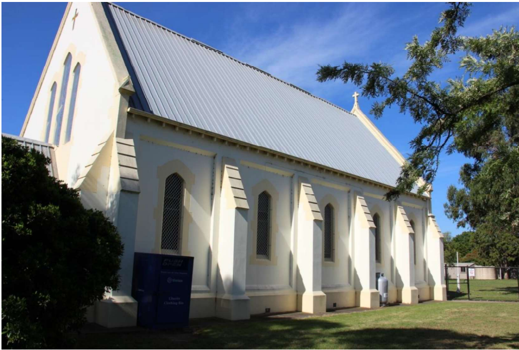
Figure D3. The south elevation. The side elevations are divided into five bays by solid buttresses. Each bay has a single window in a large recessed square panel. The windows, like those of the facade, have a pointed-arch, rendered trimmings (overpainted in a cream tone) and leadlight in pictorial and diaper-patterns, covered in modern security grill.
