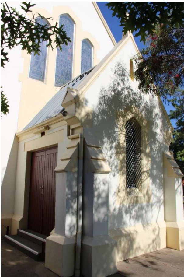
Figure D2. At the centre of the facade is the entrance porch, which imitates the details of the nave behind. The front of the porch has a pointed-arch window (covered with a modern security grill), while the sides have double timber ledged and framed doors (in a square opening) with their original handles and plates, incised with a cross.
