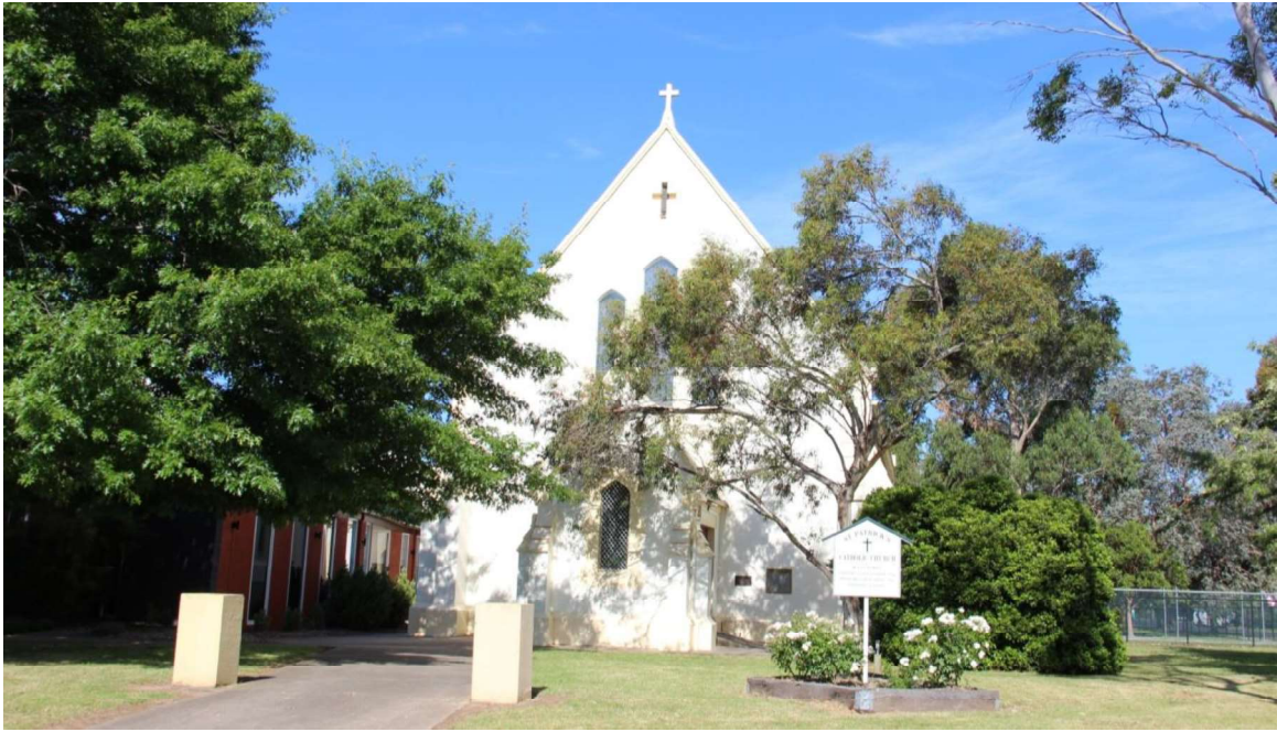
Figure D1. The church is a substantial brick structure, sitting on a large rendered plinth, with decorative render (overpainted) to the entire exterior. The steeply-pitched gabled roof is clad with (recent) metal decking with a rendered parapeted gable.
