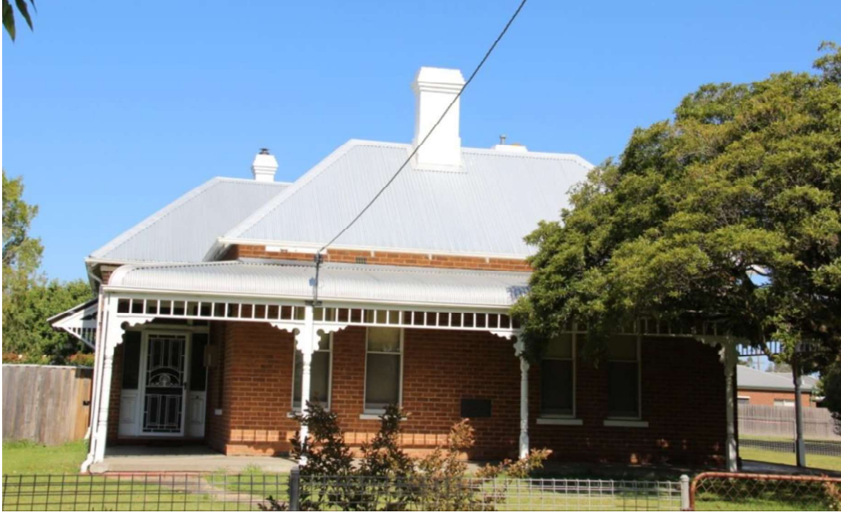
Figure D8. The 1910 rectory is a substantial brick residence with a large M-hip roof clad in (recent) corrugated iron, retaining three (overpainted) corbelled brick chimneys. A verandah with a bull-nosed profile and a concrete floor, returns on the north and south elevations, stopping at projecting hipped-roof bays.
