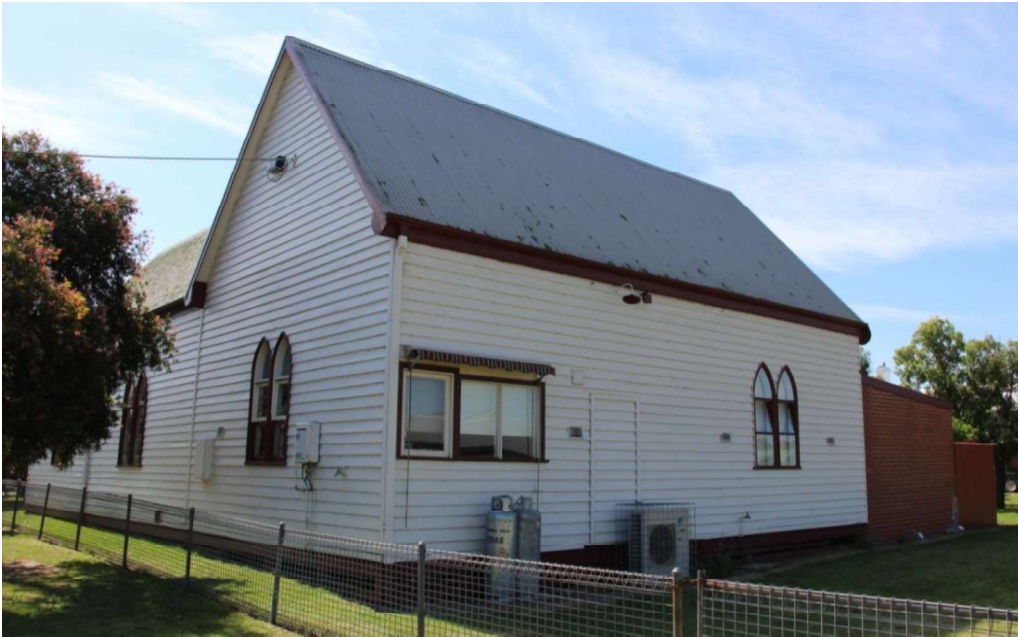
Figure D6. The east (rear) section of the hall is a weatherboard building with a transverse gable. The section contains pairs of pointed-arch windows in the same style as the 1901 building, but also has later square-headed timber-framed windows to the rear elevation.
