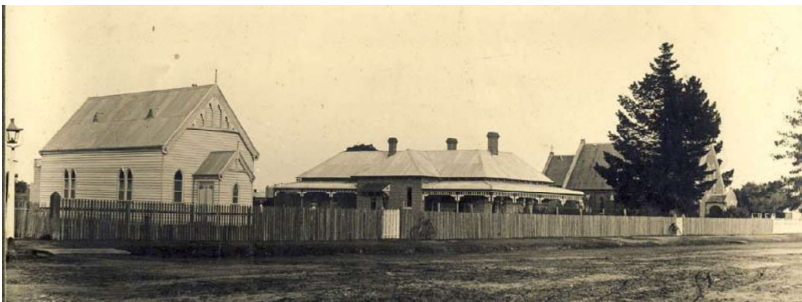
Figure H2. A photo dating post-1910 showed the complex from the north. At the north end was the timber hall with lapped corrugated iron and roof vents, and finial, in its original location, the brick rectory with lapped corrugated iron roof cladding, was central and the church was at the south end, behind a pine tree. Note the long picket fence. (SDHS).
