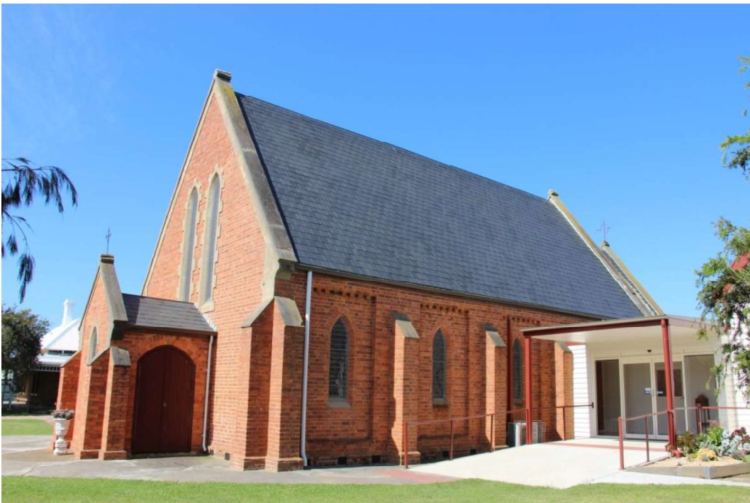
Figure D2. The south elevation. The side elevations comprise five bays, created by buttresses. Each bay has a slightly recessed panel with a row of corbelled bricks at the top. Each bay has a pointed-arch window with radiating voussoirs above and pictorial leadlight. A modern building connects part of the south elevation of the church (enveloping the two rear bays) and weatherboard hall to the south.
