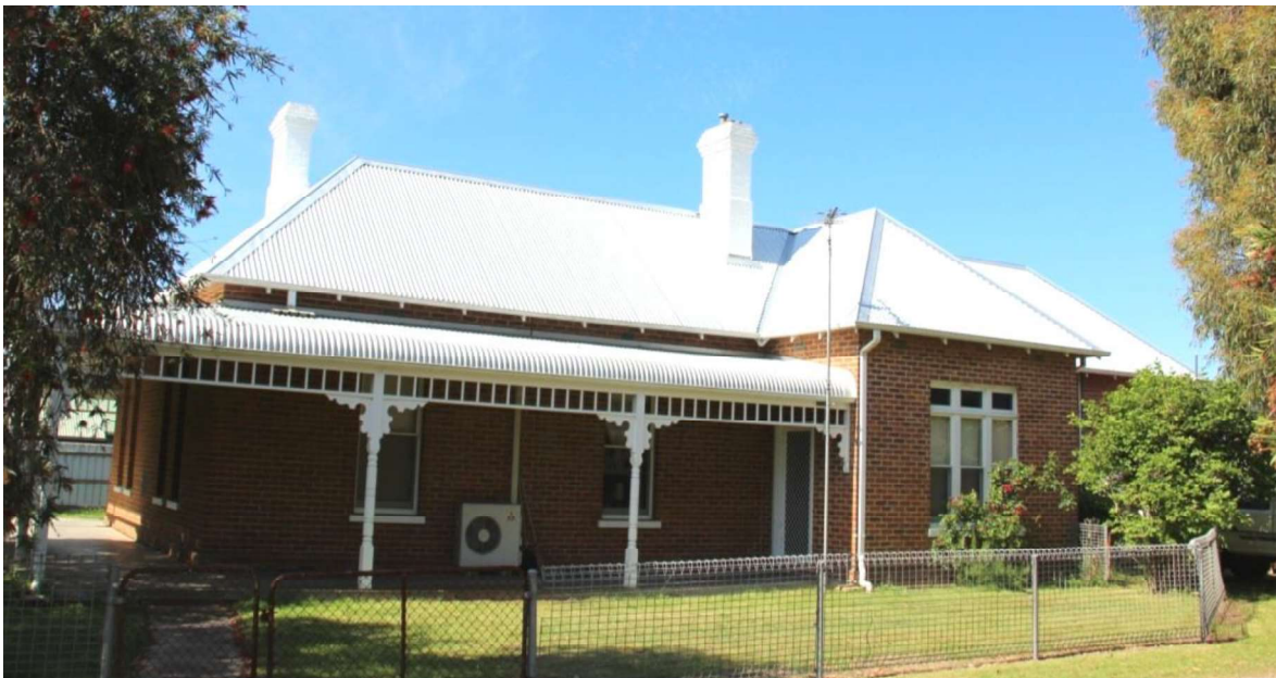
Figure D9. Windows underneath the verandah are tall narrow one-over-one sash windows, while the projecting bay on the south elevation has a large group of windows comprising three narrow one-over-one sash windows with coloured highlights. All windows have (overpainted) rendered (or stone) sills.
