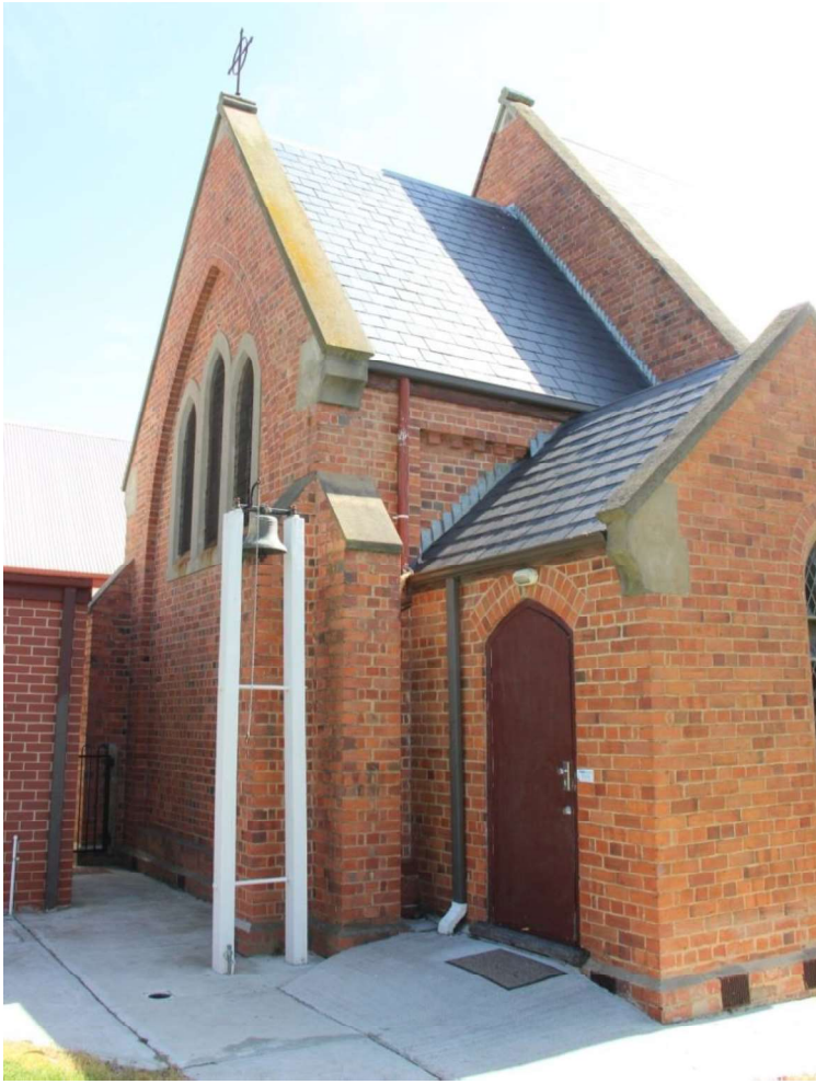
Figure D3. At the rear (east) end of the church is a large chancel (1907) with a group of three pointed-arch windows with rendered surrounds and pictorial leadlight. Projecting off the north side of the chancel is a small vestry (1907) with the same architectural details as the nave and chancel. Concrete has been built up to floor level at the doorway. A small timber bell tower stands at the rear (east end) of the church.
