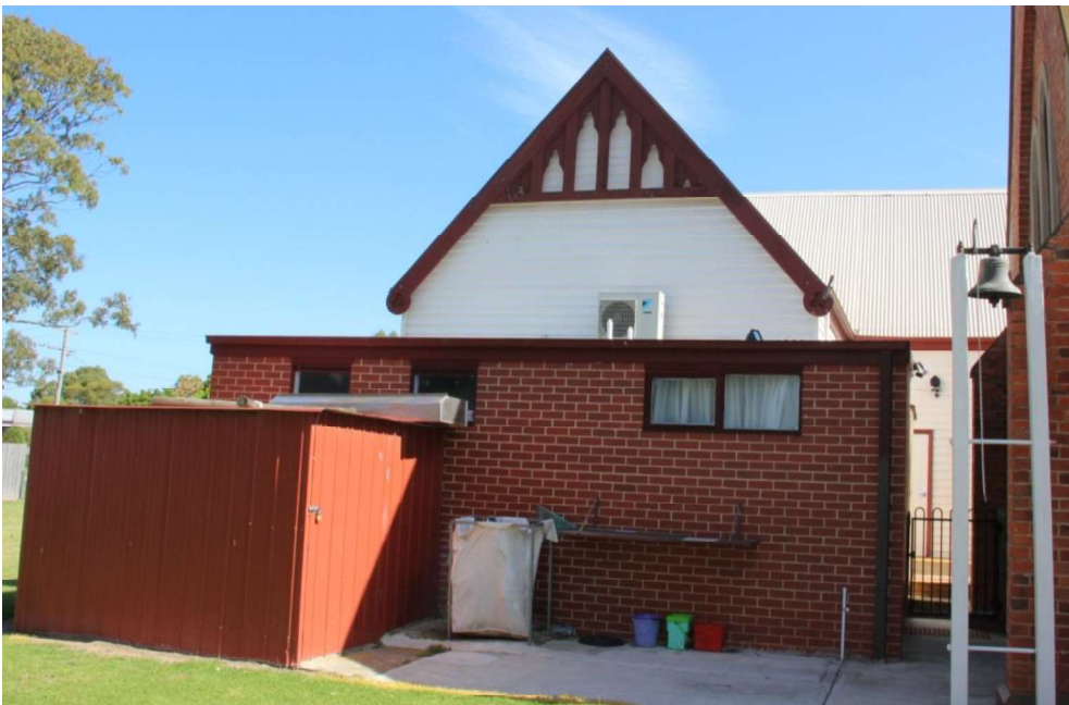
Figure D7. The gabled-end of the north elevation of the rear section of the hall retains the bargeboards and timber valance that imitate those of the facade of the 1901 hall. A modern brick addition is attached to rear of the hall.
