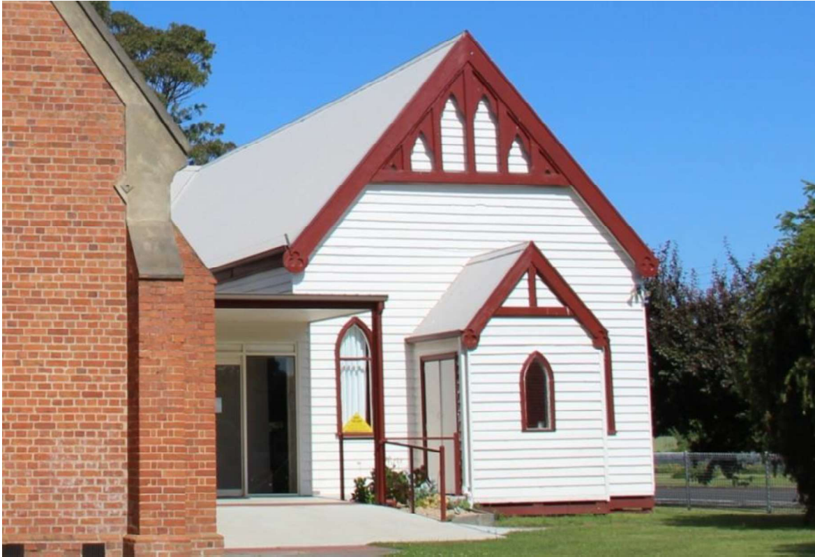
Figure D4. The 1901 weatherboard hall to the south of the church has a steeply-pitched gabled roof clad with (recent) corrugated iron, with a decorative timber valence to the gabled end of the facade. The wide bargeboards finish at the ends with lobes with a trefoil motif. A central entrance porch imitates the details of the elevation behind.
