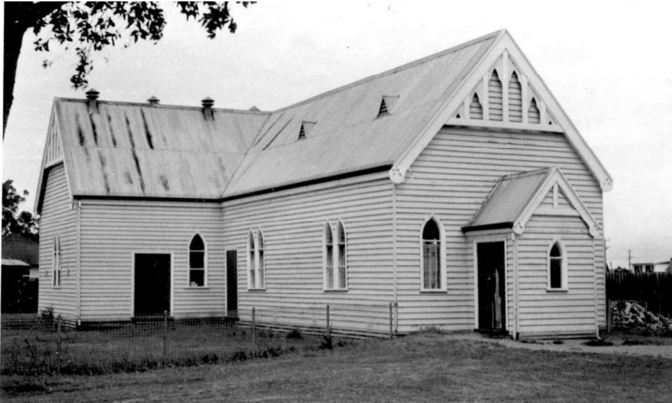
Figure H5. A photo dating to 1980 that showed the timber hall in its original location to the north of the rectory. At this date the hall comprised the entrance porch, the original gabled-roof section clad in galvanised corrugated iron, and the large transverse-gable section at the rear, projecting to the north (SLV).
