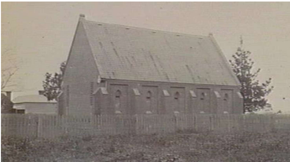
Figure H1. A photo dating between c1894 and c1907 that showed the brick church with slate roof, from the north-east, before the chancel was constructed (in 1907). To the south of the church there was a hipped-roof house which may have been the first rectory. (SLV).
