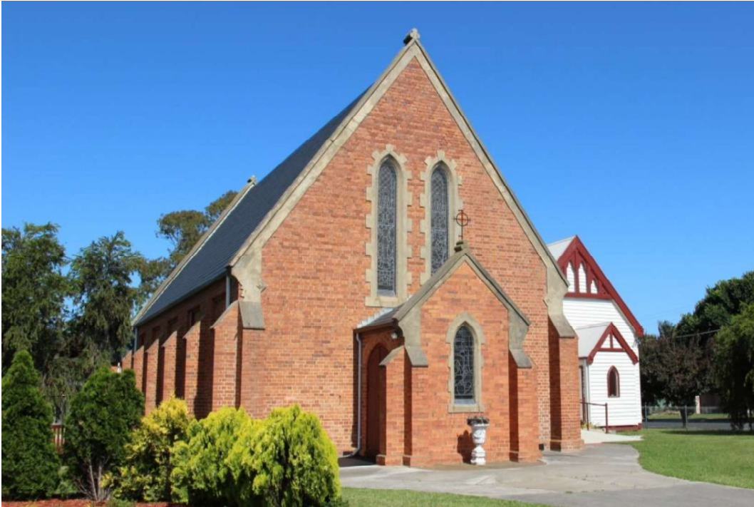
Figure D1. The church is constructed of handmade red brick in an English bond, with a small brick plinth and steeply-pitched gabled roof clad in slate. To the facade, rendered dressings (not painted) are applied to the parapeted gables, buttresses, and to the window surrounds with a quoining pattern to the sides.
