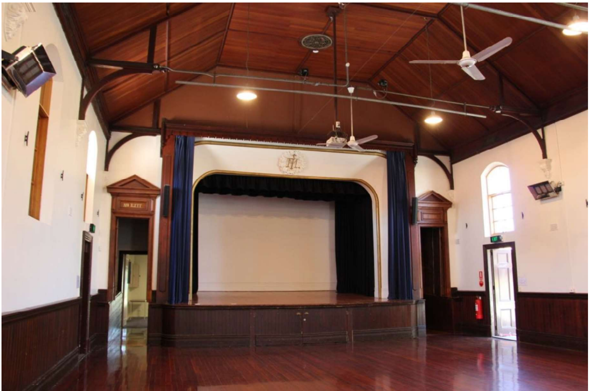
Figure D5. The interior of the hall with its original timber stage, proscenium with wreath, timber lined ceiling with cast iron ceiling rose vents, hammer beams, dado to the walls and aedicules to the original doors at the side of the stage.
