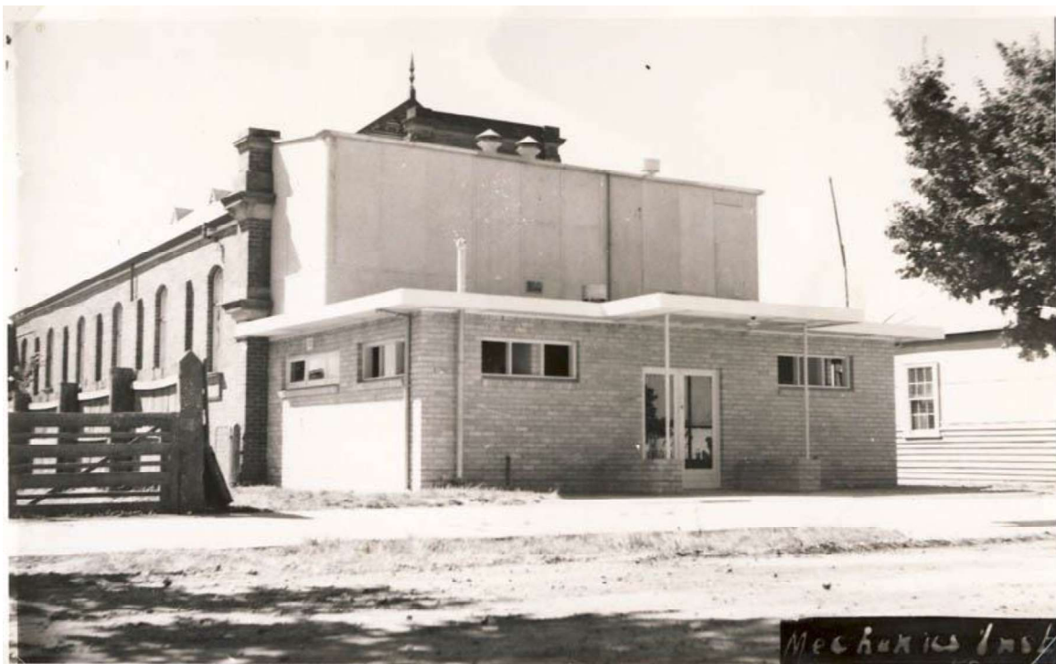
Figure H3. The hall in 1958. The front elevation had been replaced with an intrusive cream brick addition and section above, which covered the entire facade of the hall, all since removed (SDHS).
