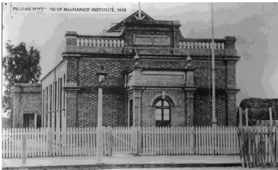
Figure H1. The hall in 1910. At the peak of the roof the gablette, flying gable end, finial and timber vents were evident, as well as the triangular vents to the roof (since removed). A flagpole stood to the right of the facade, while a timber picket fence and pedestrian gate ran along the front boundary (SDHS).
