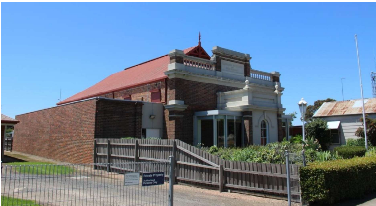
Figure D3. The west elevation of the hall is partly visible behind the modern addition. The gablette to the roof is visible, with its timber detail and finial.
