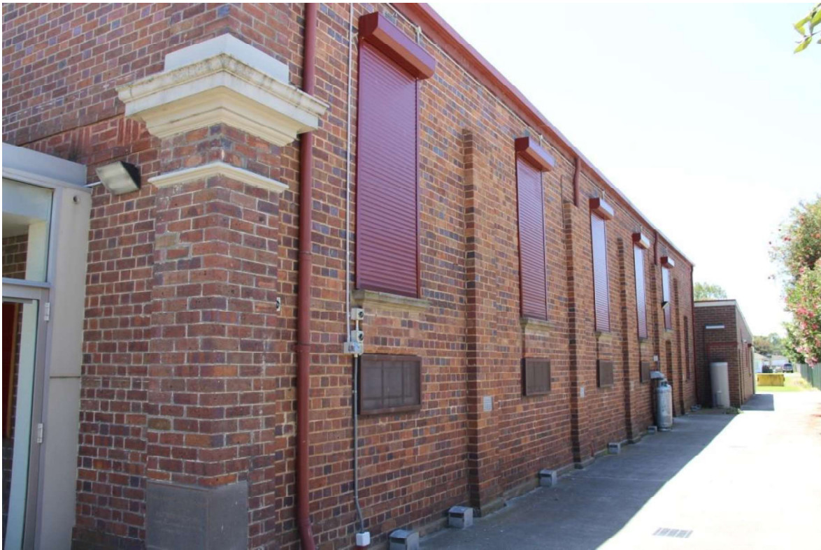
Figure D2. The east elevation with windows (behind modern roller shutters) with rendered sills and a brick apron, above a modern vent. Simple engaged buttresses are located between each window. The large modern addition to the rear extends beyond the side elevations.
