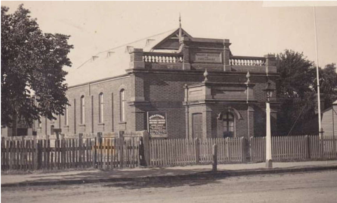
Figure H2. The hall at an unknown early date (similar to 1910 photo). At this date the roof had four triangular roof vents and the west side of the porch had a panelled entrance door (all since removed) (SDHS).
