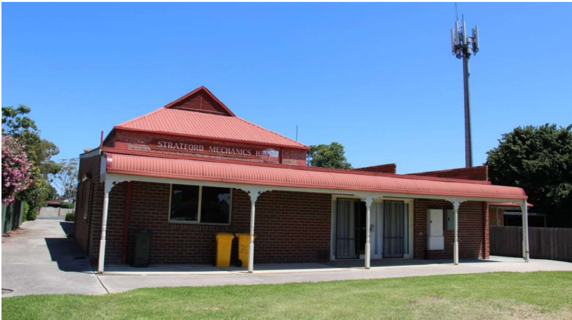
Figure D4. The rear (north) elevation with the gablette to the original section of the building, which is clad in modern metal red decking, and the lower roof-form of the modern addition, with its heritage style verandah, clad in modern red Colorbond.
