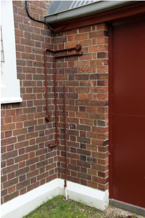
Figure D3. The entrance porch is constructed of a different coloured (lighter) handmade brick, which is keyed in to the brown brick of the nave.
