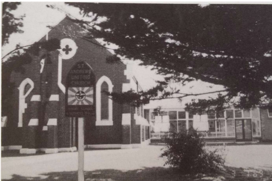
Figure H2. A photo dating to 1987 that showed the facade, with the decorative render painted bright white. The 1960s addition was evident to the east of the church and in the foreground a mature pine is partly visible (since removed; probably the large stump which remains in 2015) (Hardy 1989:96).
