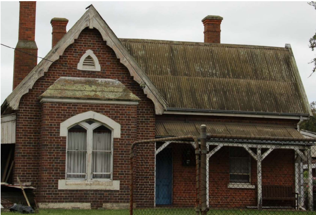
Figure D2. To the left of the facade is the brown-brick projecting gabled bay and to the right of the facade is a skillion-profile verandah clad with lapped corrugated iron, supported by timber posts with simple timber brackets.
