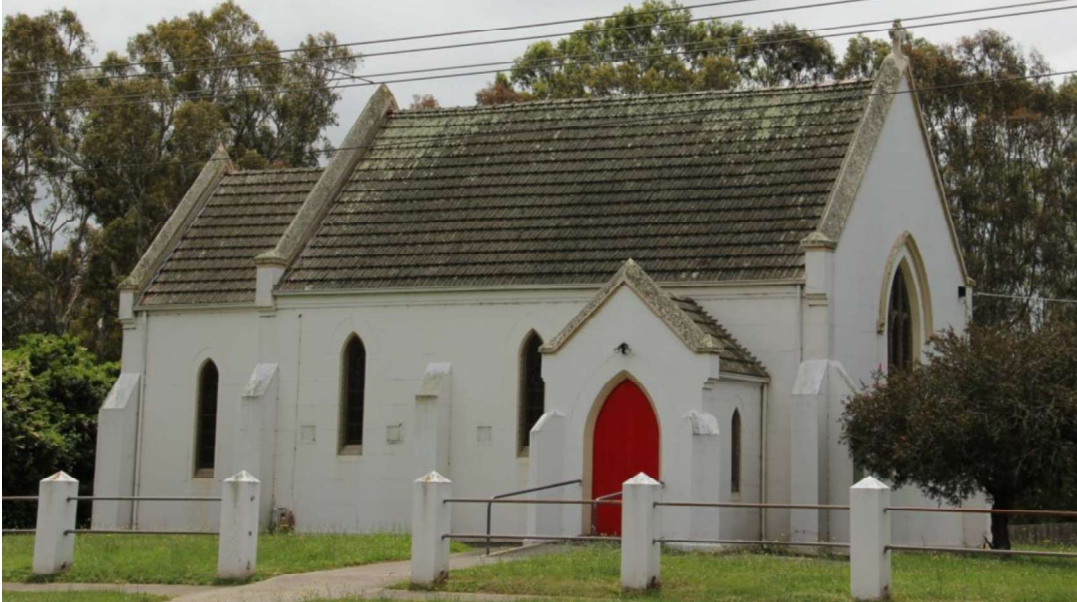
Figure D1. The church is a brick construction, with rendered walls and buttresses, with incised ruled lines to create an ashlar effect. The gabled roof is clad with (later) tiles (replacing the original slate). The entrance porch off the south elevation imitates the details of the nave, with small pointed-arch windows to the sides and a large pointed-arch opening facing south, with timber ledged and framed doors.
