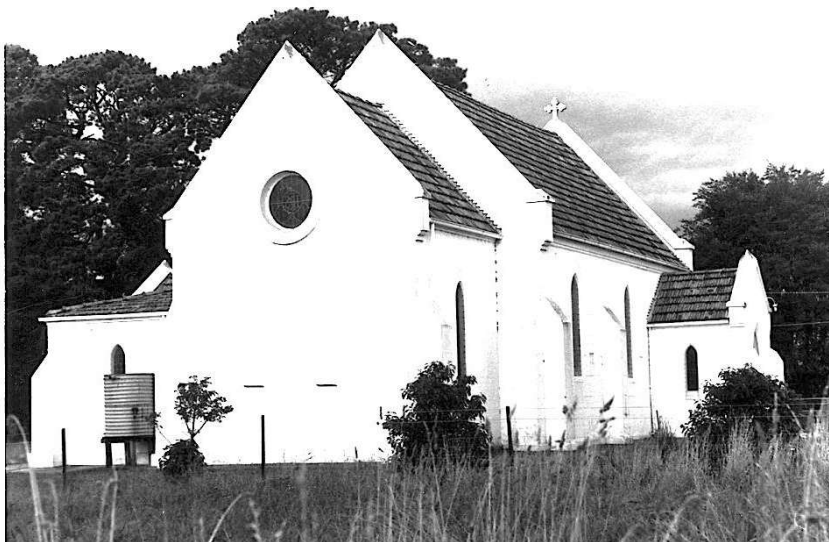
Figure H2. Photo dating to 1984, showing the (later) terracotta tiles on the roof, rear (west) end of the church. Off the chancel was the vestry and a second smaller room, all of which remain in 2015 (SLV).
