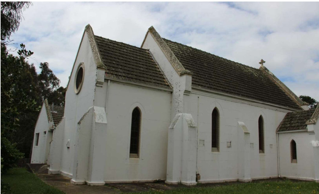
Figure D2. At the west end (rear) of the church is a chancel (constructed 1906) with a gabled roof clad with tiles and the same architectural details as the nave. The west elevation of the chancel has a large round window with leadlight to the gabled end. In the background is the sympathetic modern addition.
