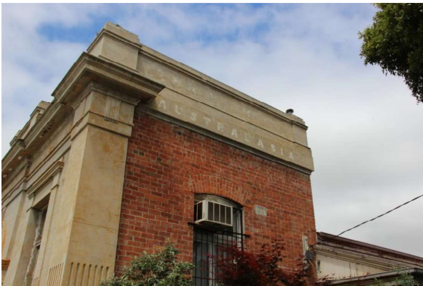
Figure D2. The west elevation of the bank, partially showing 'Bank of Australasia' and the original face red-brick wall (exposed after the chemical removal of the paint in 2010).
