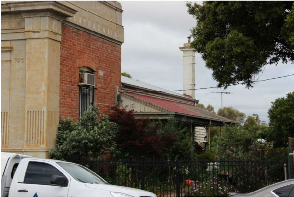
Figure D3. The west elevation showing the rendered pilaster and parapet wrapping around from the front elevation to the face red-brick wall of the bank, and the residence to the rear. The early/original skillion-roof verandah attached to the residence has been altered (cast iron brackets removed and columns replaced with simple metal pole supports).
