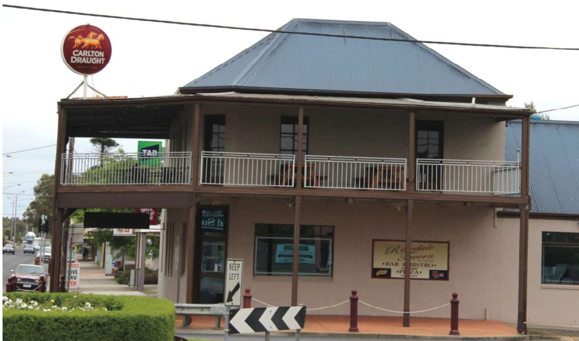
Figure D4. The east elevation is the shorter side, with two tall openings (with modern windows replacing the original French doors) to the first floor and a large opening to the ground floor (with a modern window), next to the entrance.
