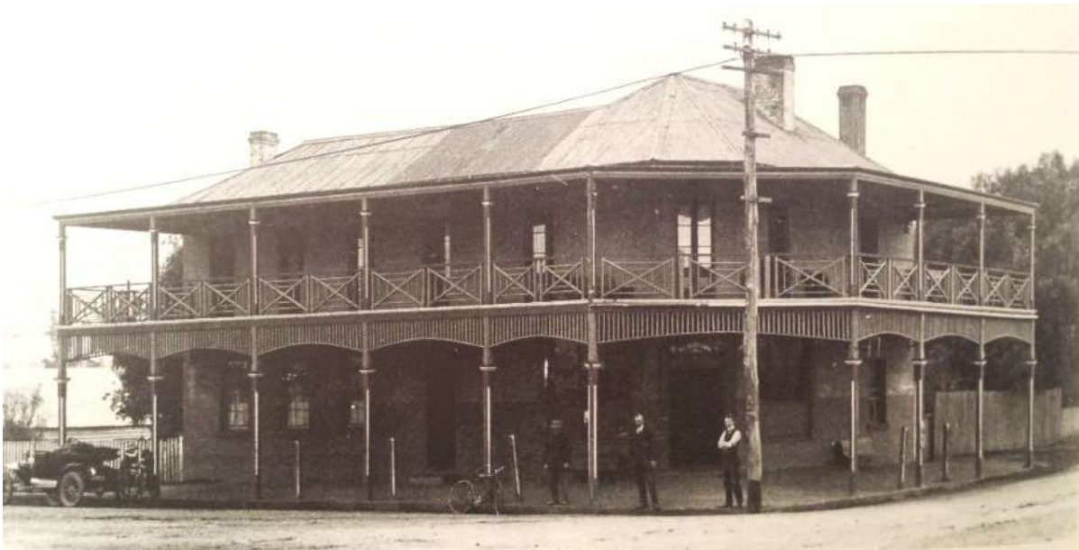
Figure H4. This photo dating to 1920 confirms that either a new balcony was constructed or that the balcony was now supported by timber posts and had a roof to the first floor. The verandah had chamfered timber post supporting both levels, with capitals and an arched timber frieze to the ground level. The cross-patterned balustrade to the first floor appears to have been retained from the earlier balcony (Hardy 1989:182). The French doors are still intact on the first floor and the walls are rendered.
