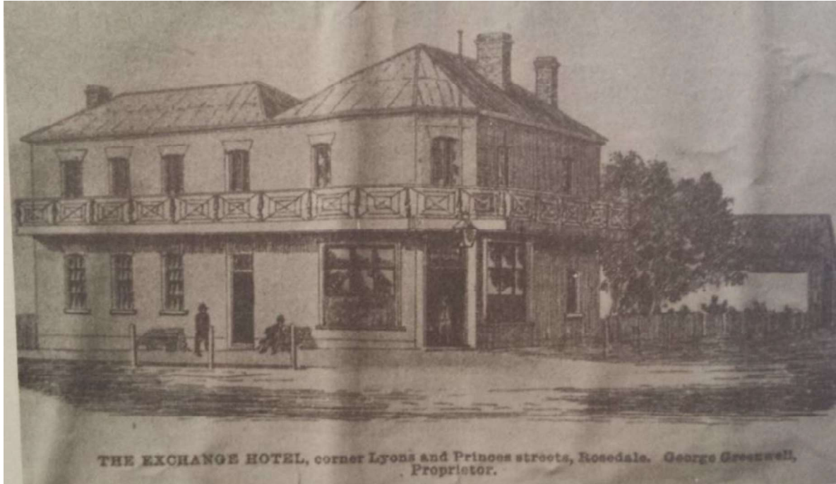
Figure H1. Drawing dating between 1881 and 1890 when George Greenwell was the proprietor. The cantilevered balcony with its cross-pattern is shown. The building looked like two separate buildings at this date (Macreadie 1989:143) and the very steeply pitched roof at the corner is intact in 2016, and may be clad in 'Morewood and Rogers' flat metal tiles in this drawing.
