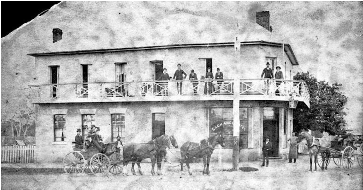
Figure H2. Photo of the hotel in 1890 showing the cantilevered balcony with its cross-pattern balustrade with turned timber posts, rendered walls, and layout of the openings of each level (Museum Victoria).
