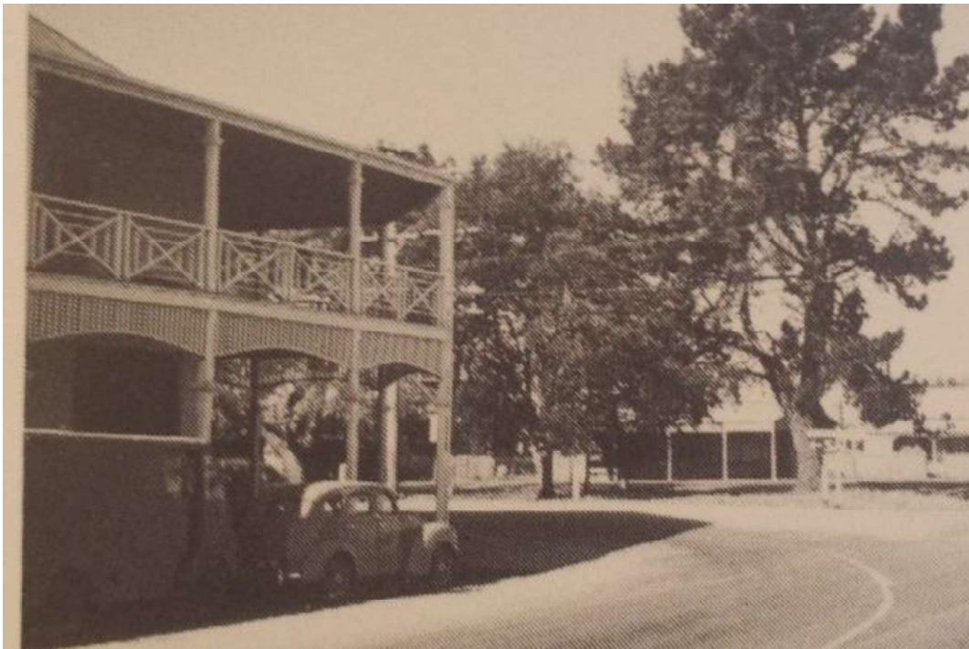
Figure H5. Photo dating to c1950 showing the corner of the hotel, looking east. At this date, the hotel retained the 1911 verandah, comprising the cross-patterned balustrade, capitals to the columns and arched timber frieze to the ground floor (Hardy 1989:590).
