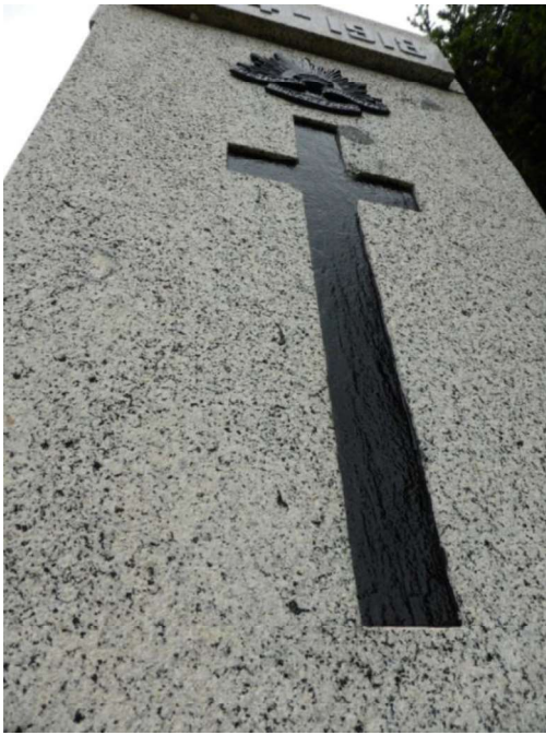
Figure D1. Detail of the polished granite of the Soldiers' Memorial, with the incised cross painted black, and metal ornament on the WW1 memorial.
