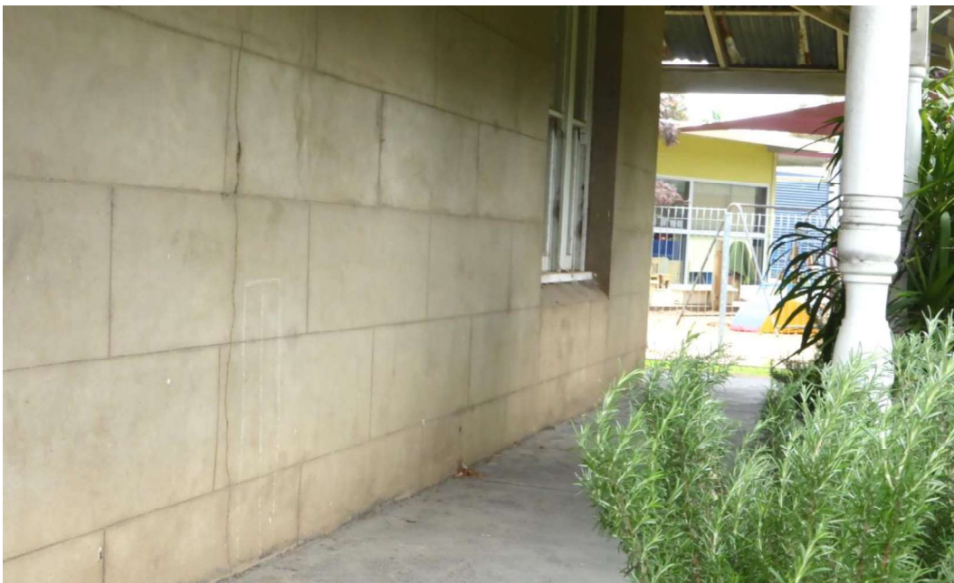
Figure D2. The walls are a concrete construction, finished with a smooth cement render that has ruled incised lines to create a large ashlar effect.
