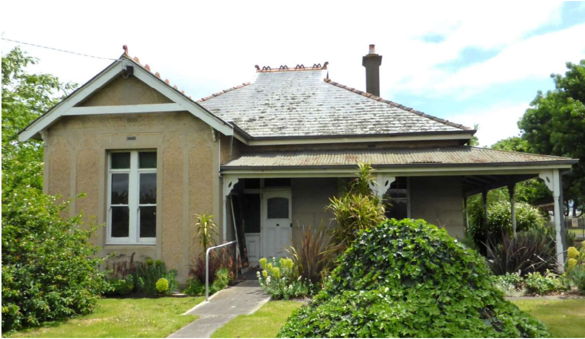
Figure D1. The 1914 concrete house fronts Lyons Street and has a hip-and-gabled roof, with gablettes to the peak (facing the sides), clad in slate with terracotta ridge cresting and gridding. The asymmetrical facade has a projecting gabled-bay to the left side that is finished with a coarse aggregate of smooth river pebbles and, in contrast, has elaborate Art Nouveau and linear details defined in a smooth render. A verandah covers the right of the facade and returns on the north and west elevations.
