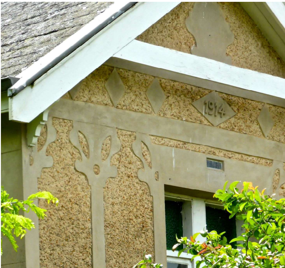
Figure D4. Detail of the elaborate unpainted Art Nouveau roughcast stucco and smooth render pattern and date of construction 1914.
