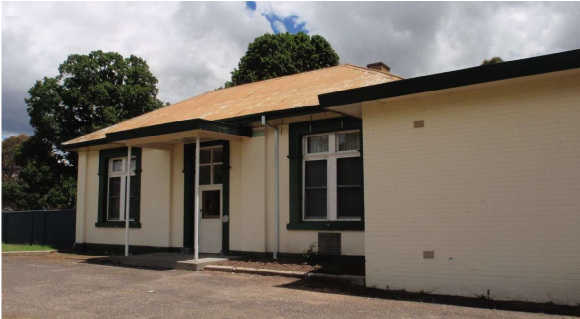
Figure D1. The original 1913 building is red brick with tuck pointing (overpainted), and rendered details, with an M-hip roof clad in corrugated iron and a symmetrical facade. Alterations include the removal of the parapet, eaves, replacement of the entrance door and highlights, addition of an unsympathetic entrance porch and a 1961 addition to the north elevation.
