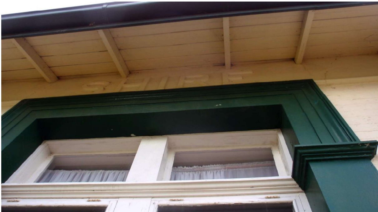
Figure D2. The words 'Shire Hall' and the date '1913' remain in raised letters beneath the 1961 eaves. The entrance and flanking windows are framed with original wide pilasters and sills (all overpainted in a heavy green colour). The eaves are from the 1961 changes, but the windows are original.
