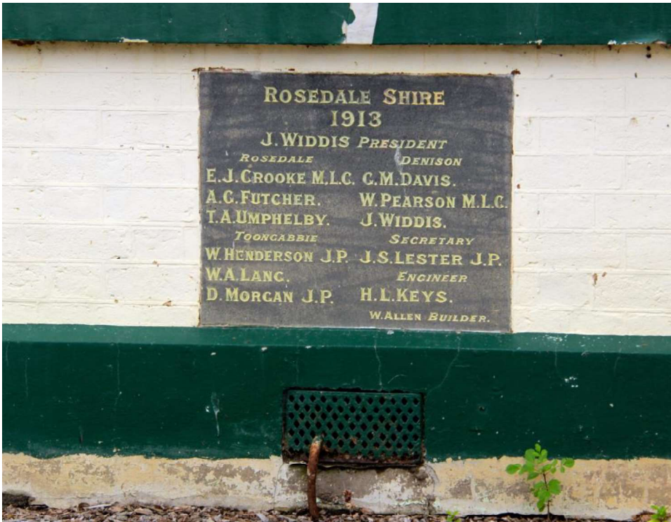
Figure D3. The 1913 Foundation Stone with hand cut incised and gilded lettering has remained intact. The raised lines of the tuck pointed can be seen under the white paint. The dark green coloured render was originally unpainted.
