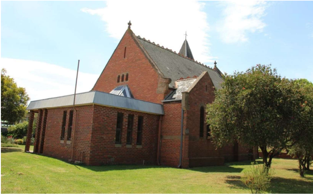
Figure D5. The rear (north-west) elevation of the church showing part of the roofline of the 1904 bay window, concealed (or removed) by the post-1970s flat-roofed addition. Projecting off the south-west (side) elevation is a small vestry, with the same architectural detail as the 1904 nave.
