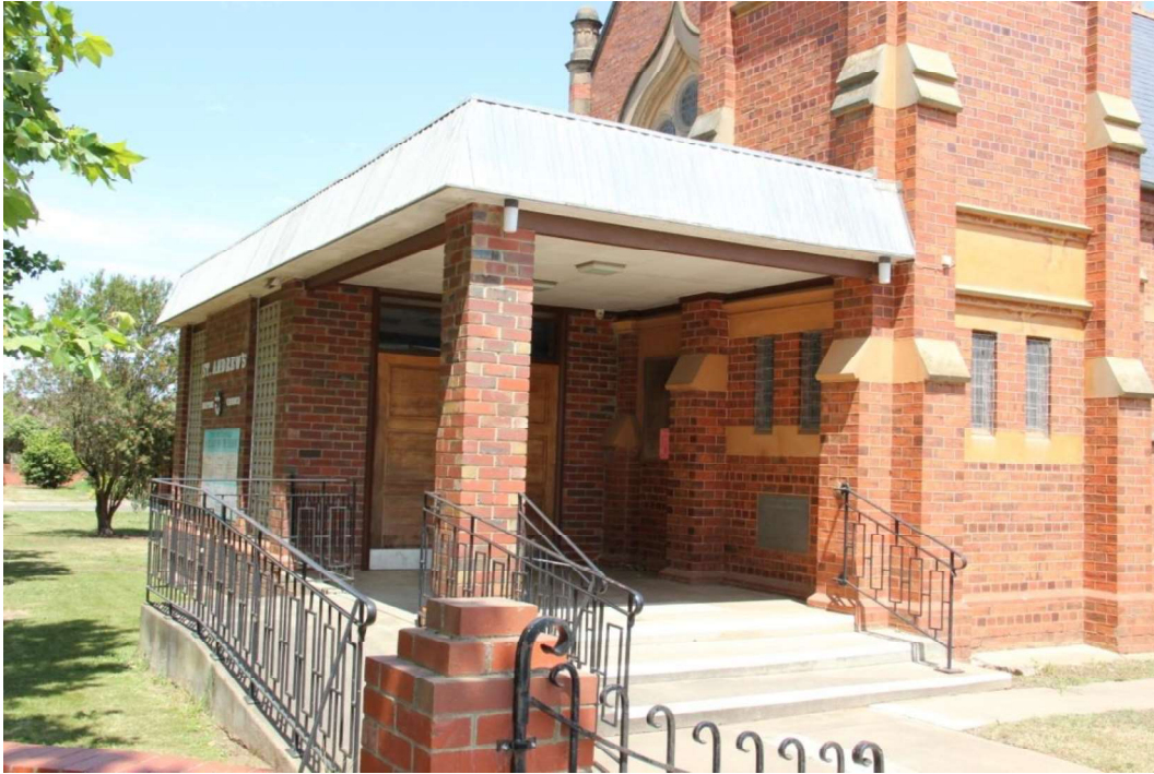
Figure D3. The original entrance porch was removed and replaced with a modern flat-roofed brick entrance porch and foyer, post-1970s. A modern concrete ramp and stairs lead to the entrance with a metal balustrade.
