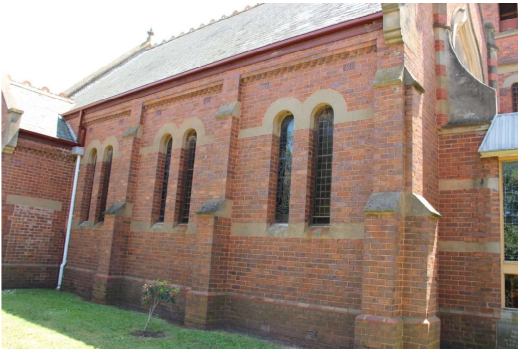
Figure D4. The side elevations are broken into four bays by buttresses with rendered coping. Each bay holds a pair of tall, narrow round-arched windows with (pictorial or geometric) leadlight. Pictured is the south-west elevation, with the vestry to the rear.
