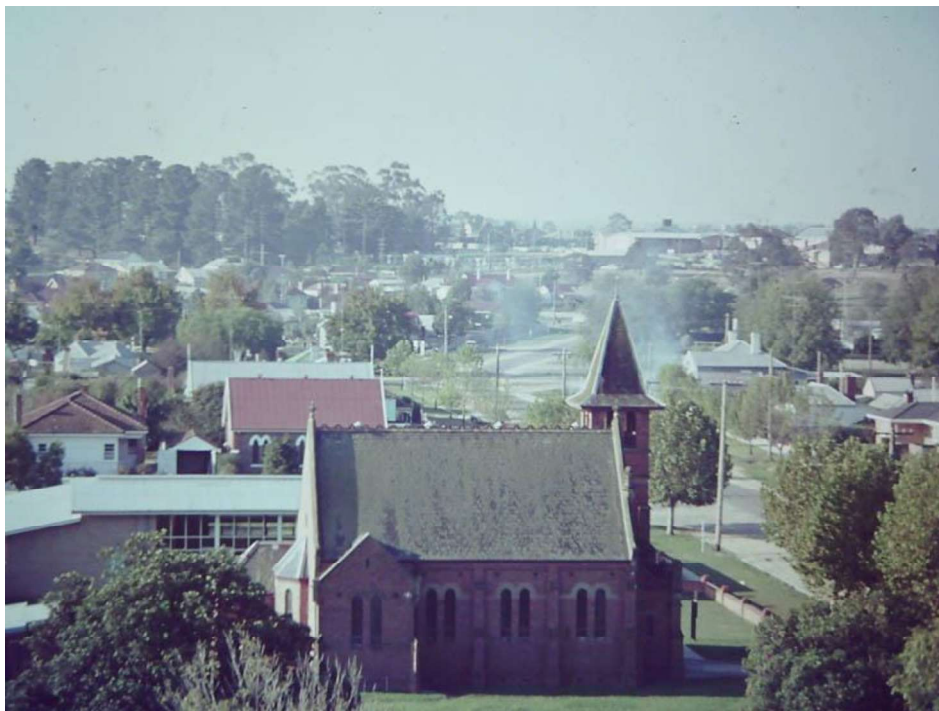
Figure H4. A photo dating to the 1970s that shows the south elevation of the church. The rear of the church had a small bay window (the roofline of which is still evident in 2015 above the later addition) and small vestry projecting to the west (remains as part of a later extension). The picket fence has been replaced with the brick one (MDHS, ID. P04962VMFF 1970s).
