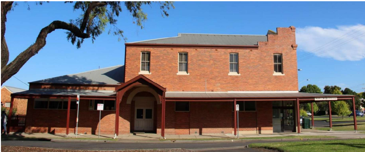
Figure D3. The parapet to the facade steps down on the side elevations, revealing the hipped roofline (with a gablette facing north), particularly from Foster Street. The first floor retains four original two-over-two sash windows with radiating voussoirs above and rendered sills.
