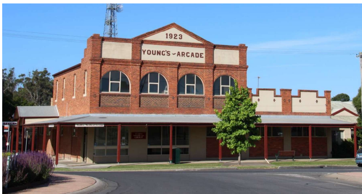
Figure D1. The two-storey red brick building faces Johnson Street and has a tall parapet and pediment with rendered panels and the words '1923' and 'Young's Arcade' in relief. To the east
