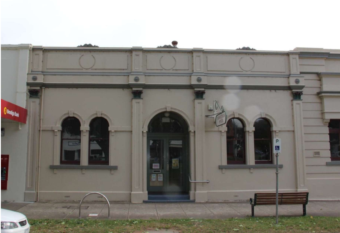
Figure D1. The facade of the Mechanics Institute (1886) with its smooth-rendered (overpainted) facade with Classical details and semi-circular arched openings.
