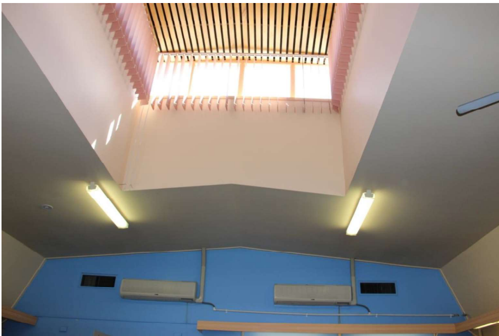
Figure D5. The clerestory windows of the room to the left of the entrance, in the 1922 World War I Hall.
