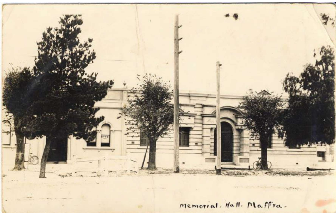
Figure H2. To the right is the Great War Peace Memorial Hall in 1923-4, soon after it was built. Note the polished granite columns had not yet been installed at the entrance at this date. To the left is the 1886 Mechanics Institute (MDHS, ID. P04278VMFF).
