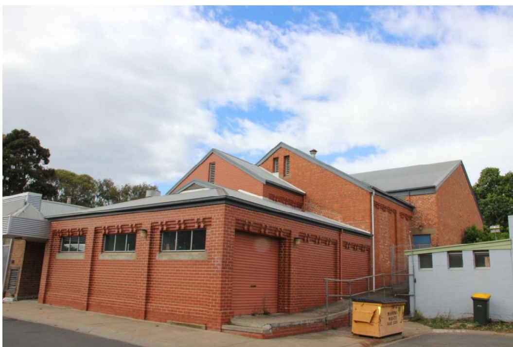
Figure D9. The transverse gable section of the 1925 hall, followed by the sympathetically designed additions dating to the 1990s.
