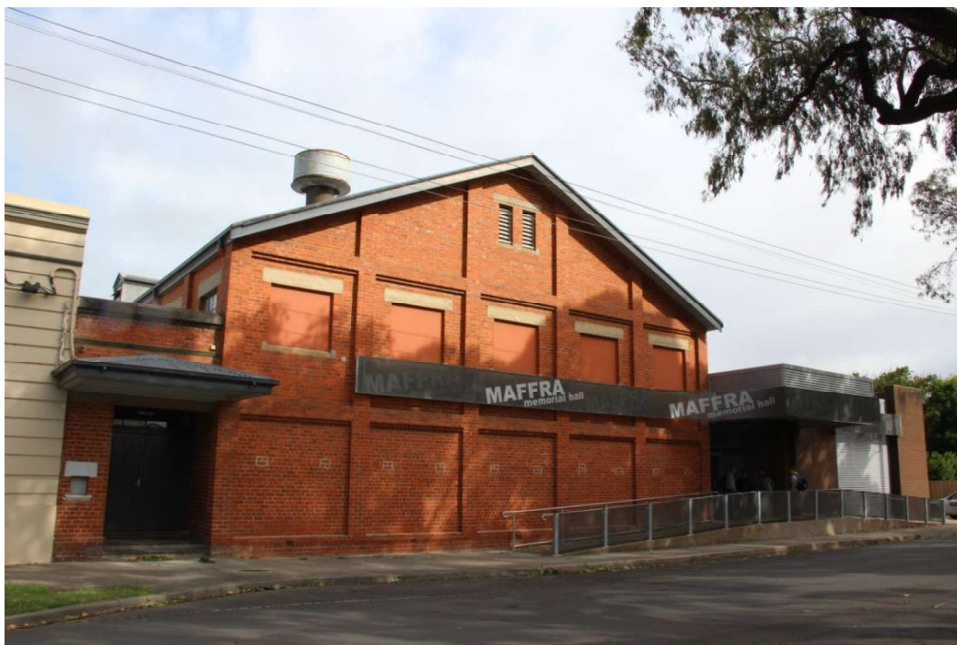
Figure D8. The 1925 Soldiers' Hall fronting Foster Street. The inter war stripped classical style building is a substantial red-brick construction with the gabled-end and façade broken up into panels by horizontal and vertical rows of corbelled bricks
