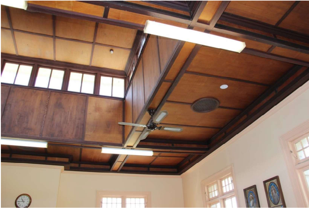
Figure D4. The unpainted timber paneling of the ceiling and clerestory windows of the RSL club room in the 1922 Great War Peace Memorial Hall.
