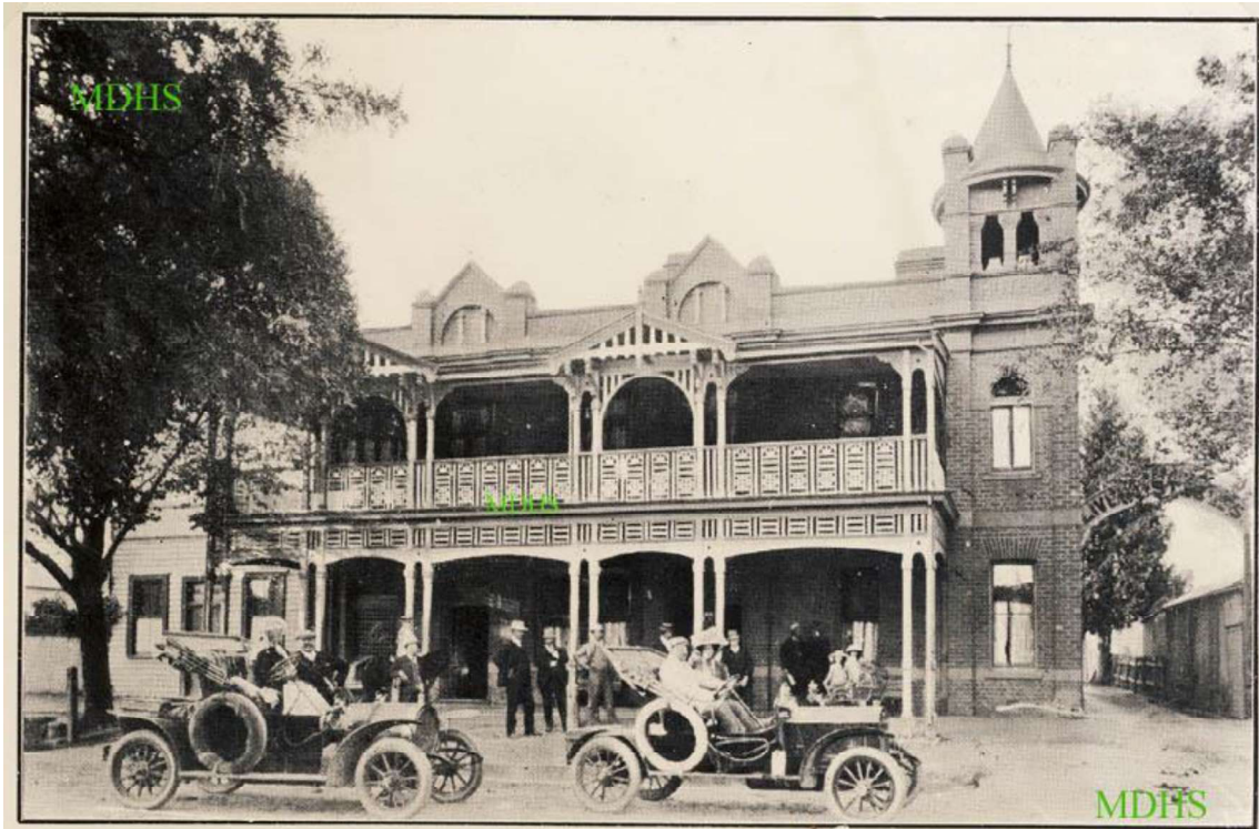
Figure H2. A photo dating to 1915 that showed the facade of the two-storey hotel. To the right of the tower was an arched structure above a side lane (removed) (MDHS web).
