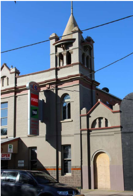
Figure D2. At the southern end of the facade is a tower that finishes above the parapet with a candle-snuffer roof (with a flagpole or very tall finial), supported by four corner piers which extend above the roof. Below the parapet, the tower has a round-arched window (with a later
