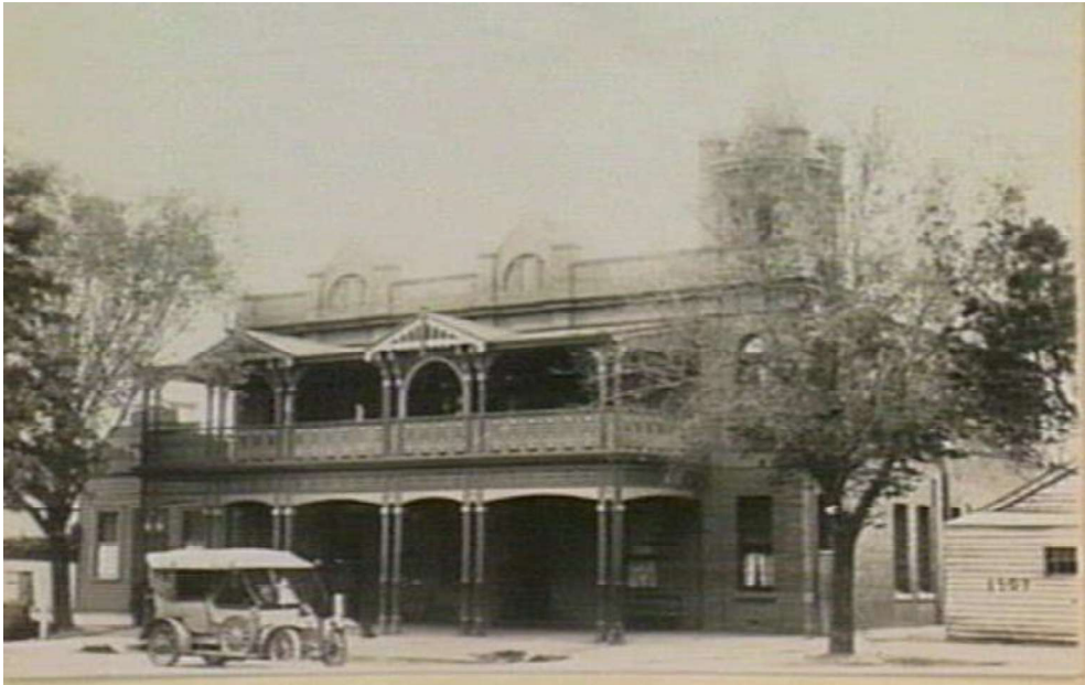
Figure H3. A c1915 photo shows the hotel and part of the east elevation. The photo showed the square-headed windows to the ground floor of the side elevation (SLV).
