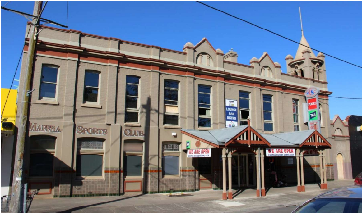
Figure D1. The facade has a smooth render to the ground floor and tuck pointed brick to the first floor and parapet (the entire facade is overpainted). The ground level has a c1930s tiled dado, in green, grey and orange glazed tiles. The facade is divided into narrow bay by engaged pilasters that extend from ground level to the parapet.
