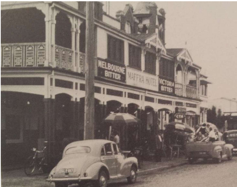
Figure H4. This c1940s or 50s photo showed a detail of the original verandah in closer detail. The frieze had been removed from the ground level by this date, but the timber valences that were positioned below remained. The exterior of the ground floor had been tiled (the lower portion) by this date (Pearce 1991:15).
