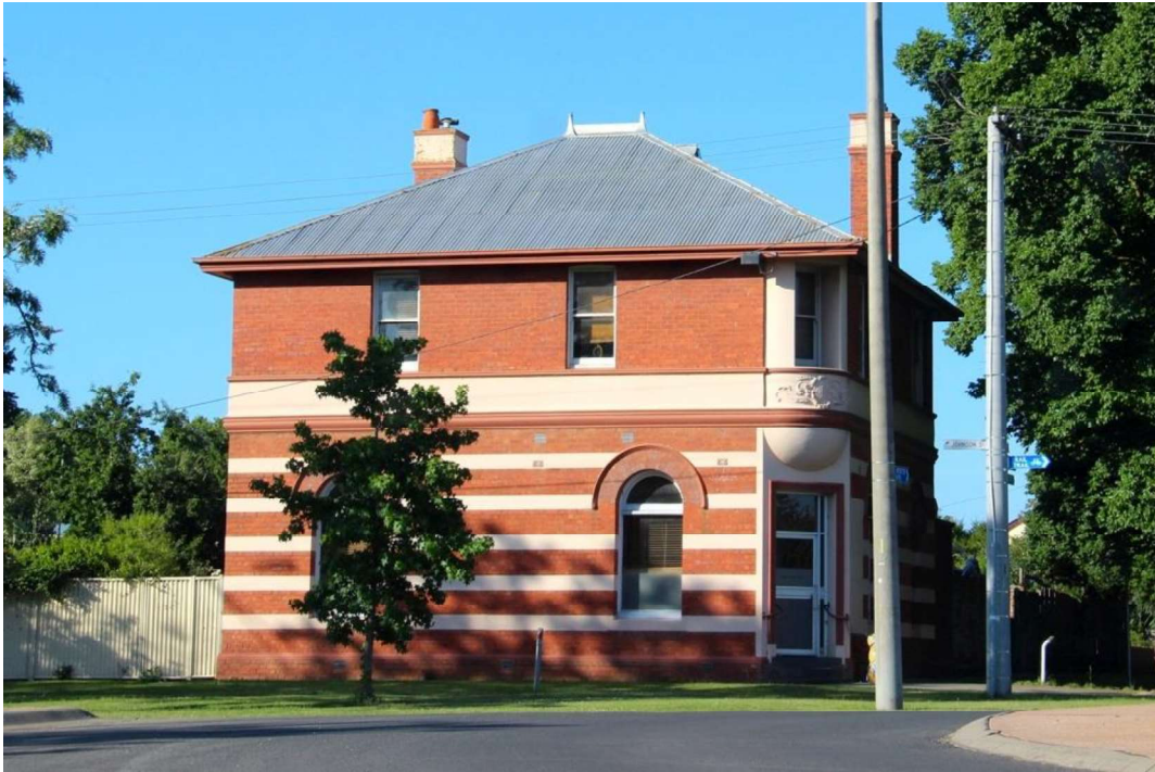
Figure D1. The Johnson Street elevation with the chamfered corner entrance and projecting oriel balcony.
