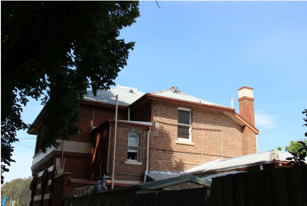
Figure D3. The rear elevation constructed of brown brick (not tuckpointed), and the northern roof faces with the triangular roof vents. The hipped roof of the single-storey portion of the building is evident; the tall corbelled-brick chimney is just out of frame to the right.
