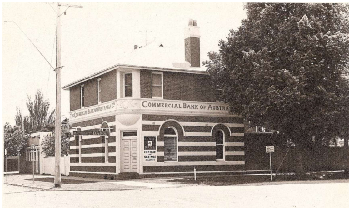
Figure H4. The bank at an unconfirmed date, when it still served as the Commercial Bank of Australia (pre-1990s). It illustrates that by this date the bank had painted rendered decoration (MDHS, ID. P02055VMFF).
