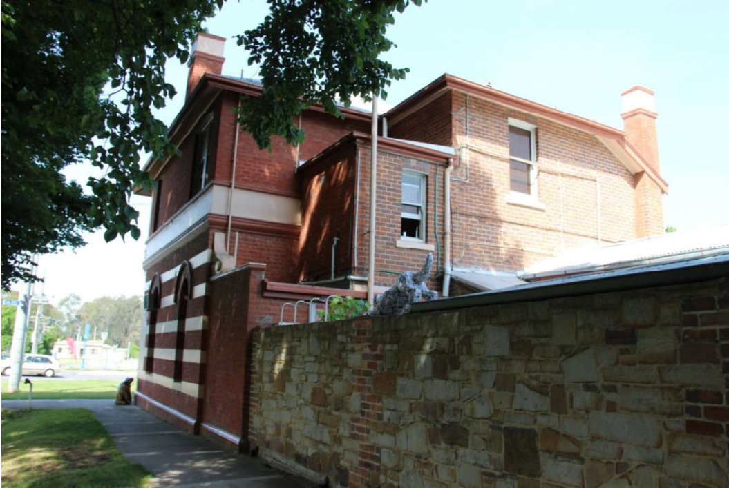
Figure D5. The rear (north-east) elevation. This boundary comprises the original tall red-brick wall with rendered scroll bracket, and the post--2000 sandstone wall with red brick quoins.
