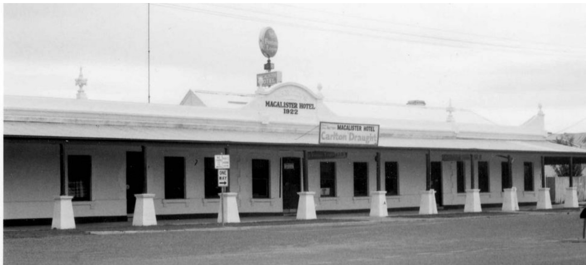
Figure H5. This 1979 photo showed the facade without the weatherboard room at the west end and the verandah that now continued, supported by similar posts and piers (SLV).
