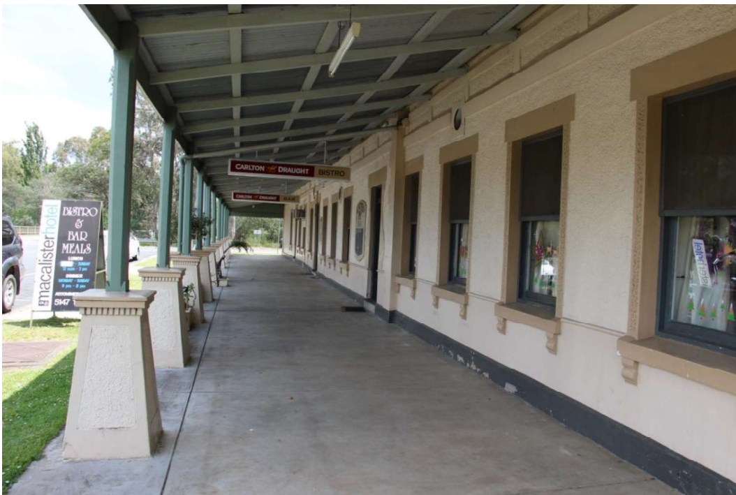
Figure D3. The facade has a rendered plinth at the base. The bottom quarter of the wall has smooth render, while the top section of the wall has rough-cast render. The verandah is supported by stop-chamfered timber posts on large tapered piers (in the shape of a battered pylon, reflecting
