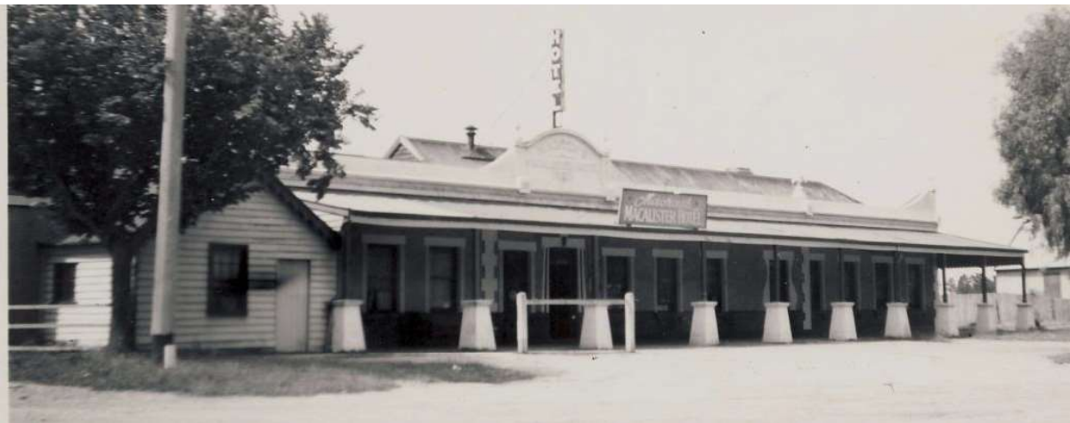
Figure H3. A pre-1965 photo. The facade of the hotel, with the small weatherboard room at the west end of the facade is visible. A sign erected on the verandah read 'Macrae's Macalister Hotel' and a tall 'Hotel' sign was stood behind the parapet. The gable and hipped roofed building behind the 1922 new plaster on the façade is likely to be part of the 1863 building (MDHS, ID. P03710VMFF).
