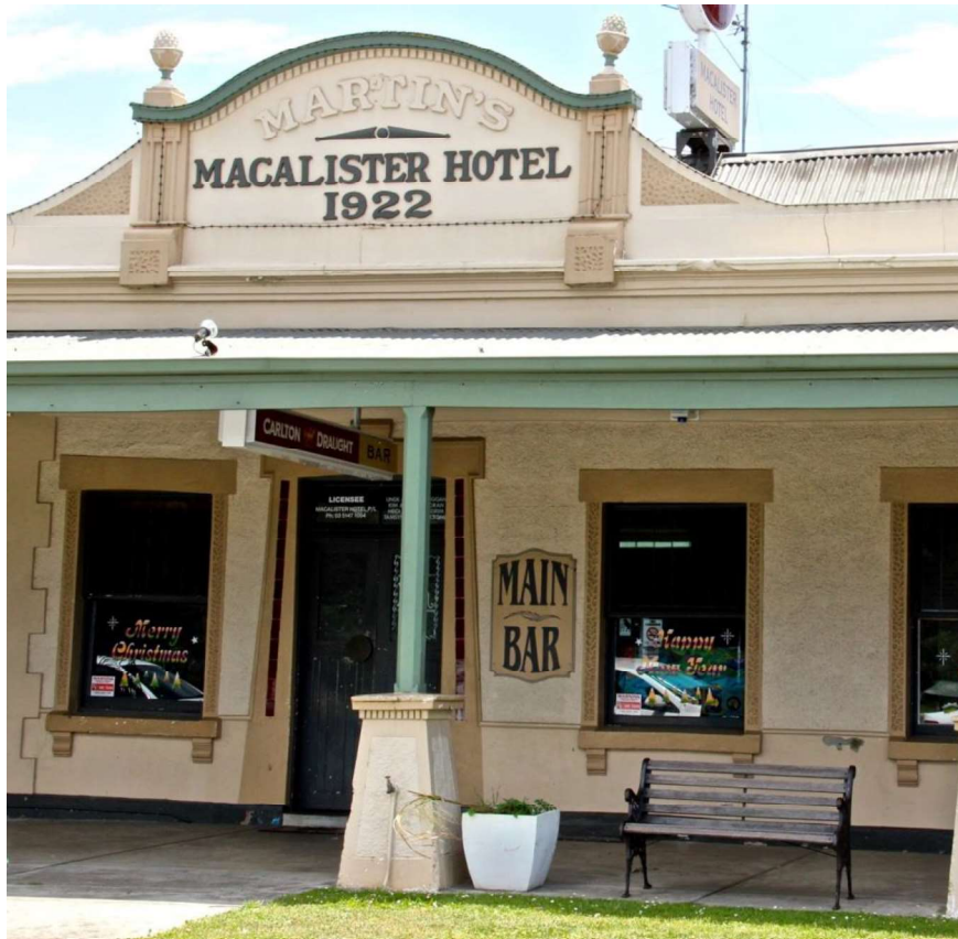
Figure D2. The ornate central parapet read's 'Martin's Macalister Hotel 1922' in relief. Behind the parapet, the gabled-roof of the (possibly c1863) building behind is evident. Beneath the verandah, this join in the building is marked by a vertical band of smooth rendered quoining.
