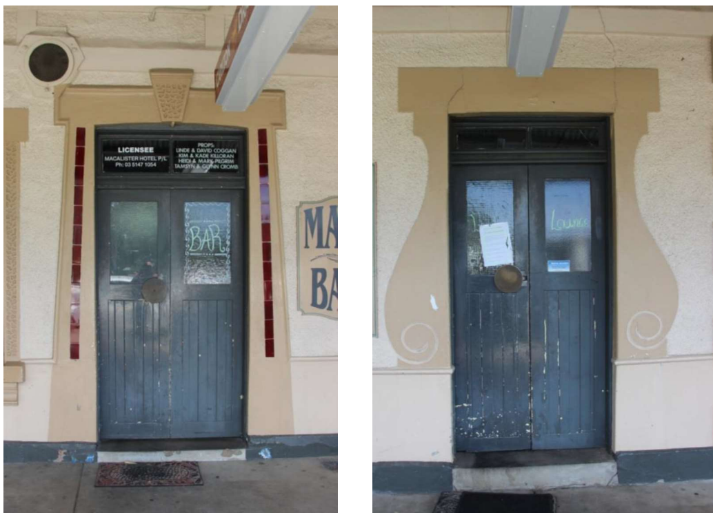
Figure D4. The surrounds to the doors of the facade are varied and elaborate. The main entrance has an Egyptian styled entrance comprising a rendered lintel, a bold keystone with vermiculation and tapered sides with a vertical line of red glazed tiles. Other entrances have a surround with a rendered lintel which extends to the sides in large lobed pattern at the base.
