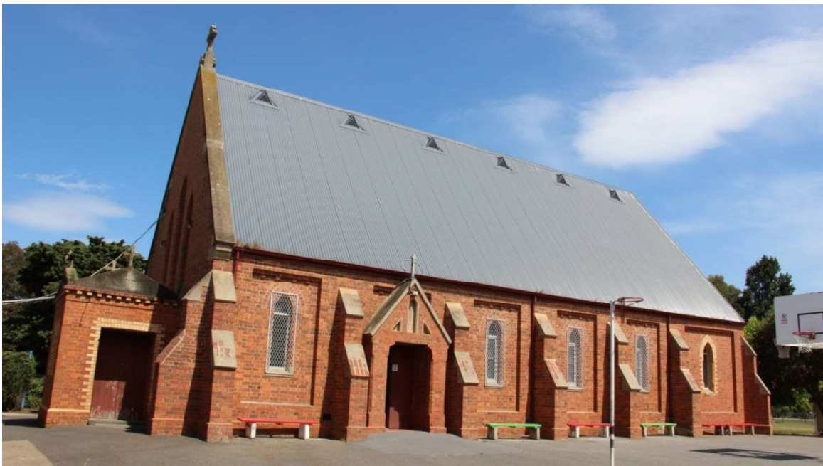
Figure D2. The east elevation. The side elevations are broken into five bays by wide two-tiered buttresses with rendered coping. Each bay has a recessed panel, with corbelled bricks to the top,
