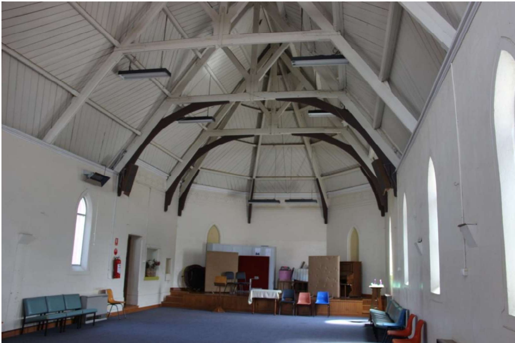
Figure D6. The interior of the church is overpainted in white, including most of the exposed timber roof trusses. The ceiling is lined with timber boards. A band of quatrefoil decoration remains at the top of the walls at cornice level. The walls are incised with ruled lines, to create an ashlar effect.
