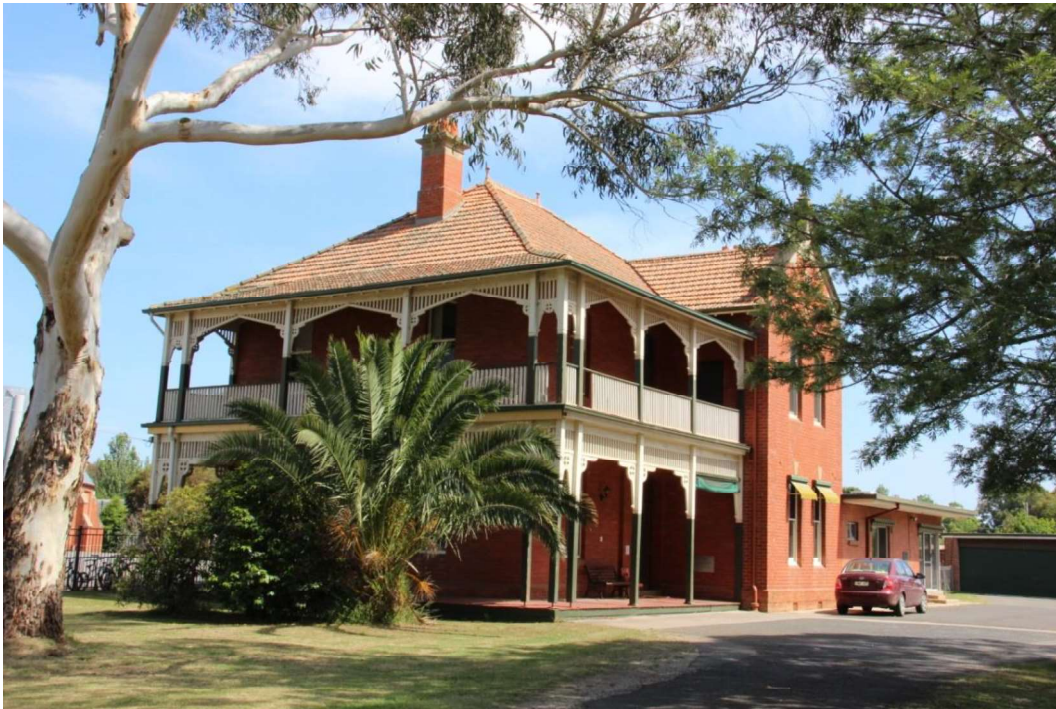
Figure D7. The large two-storey red brick building has a hip-and-gable roof clad in terracotta tiles with decorative ridge cresting and three brick chimneys with rendered caps and two terracotta chimney pots.
