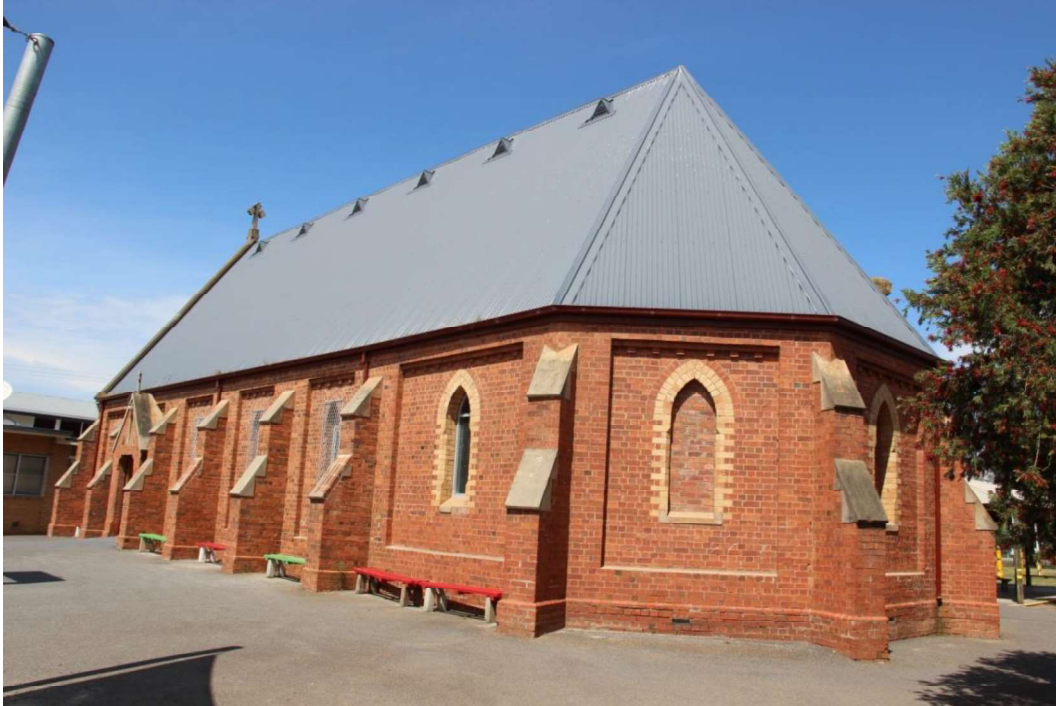
Figure D5. At the north (rear) end of the church is a chancel bay (1893) with a hipped roof, forming four bays to the exterior. The chancel imitates the recessed panels of the side elevations of the 1871 nave, but has cream-brick details to the windows like the porch and vestry (also 1893).
