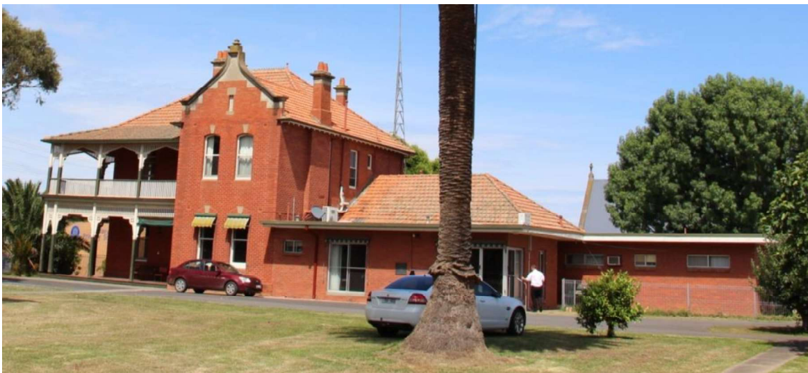
Figure D8. The verandah stops on the east elevation when it meets the two-storey bay with an ornate Flemish gable with rendered dressings. Off the north elevation is a single-storey addition (which is primarily a later addition).
