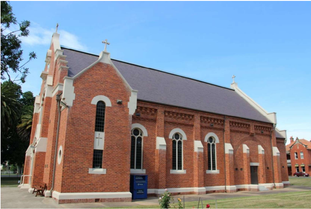
Figure D11. The projecting bays to the side elevations (immediately behind the facade) have rendered parapeted gables with crosses to the peak, and roofs clad in slate. The main faces of these bays have very tall narrow semi-circular arched window with leadlight.
