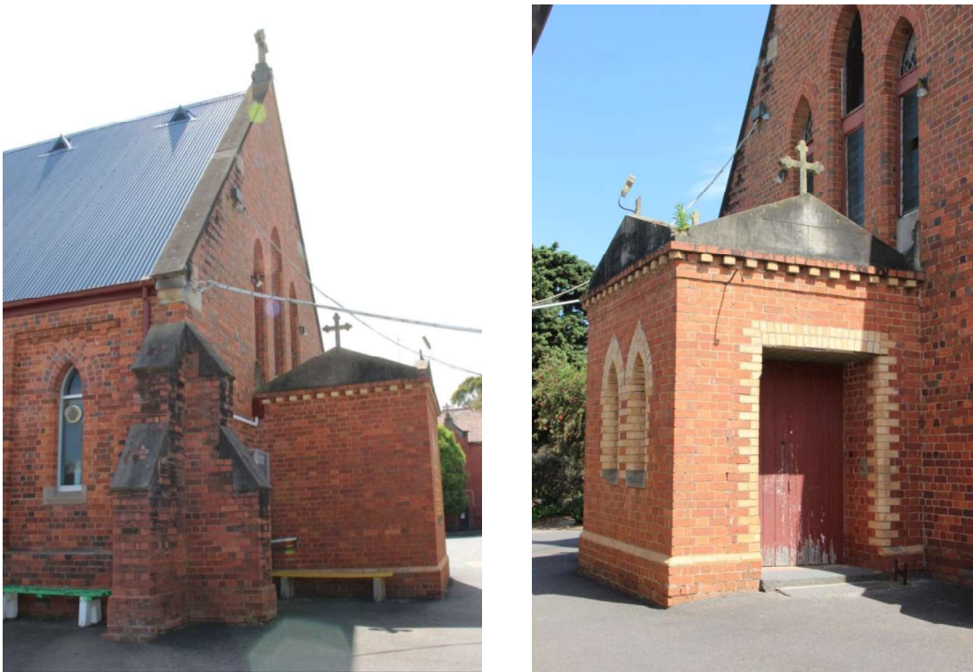
Figure D1. The facade and the west (left) and east (right) side of the porch. The church is constructed of handmade red bricks in an English bond, with a brick plinth and a steeply-pitched gabled roof clad in recent Colorbond. Central to the facade is an entrance porch (1893) with rendered pediments to each face (incised with ruled lines to create an ashlar effect), with crosses to each peak.
